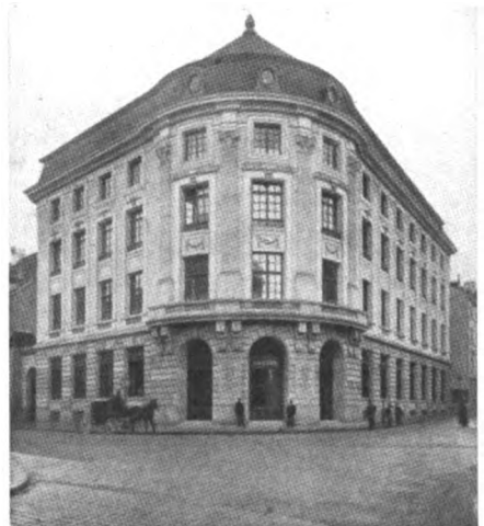
Basle Office Swiss Bank Corporation
