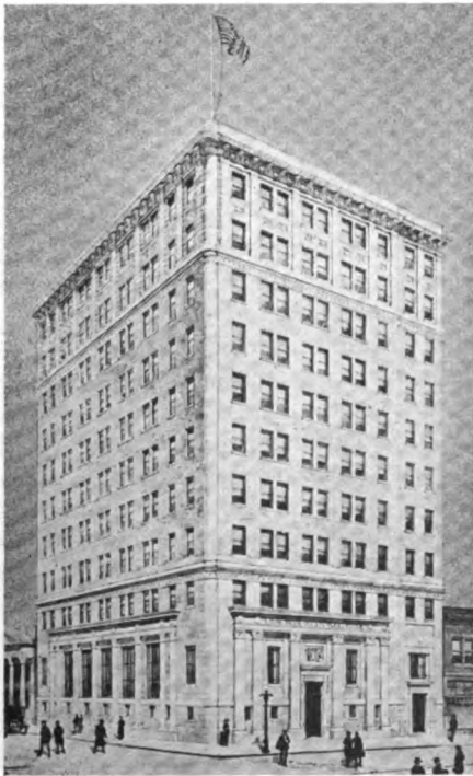
Ouachita National Bank, Monroe, La., a bank building in one of our smaller cities that in the beauty of its architecture equals the best structure in any community. It is now being built by the Underwood Contracting Corporation.
