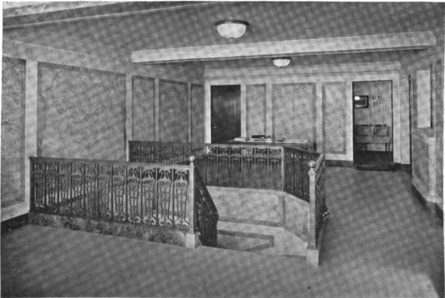
Stairway Leading to Safe Deposit Vaults, National American Bank of New York
