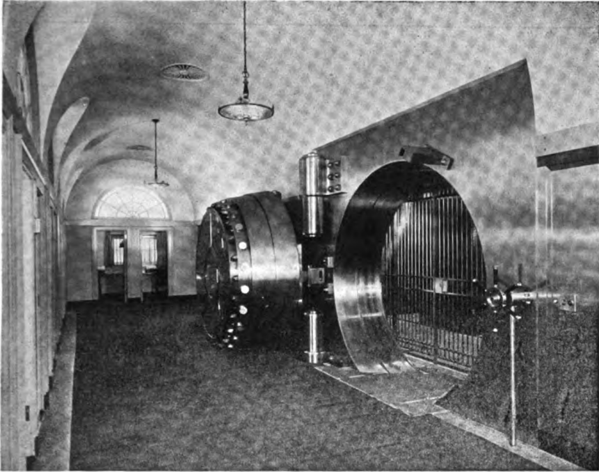
The new safe deposit vaults of the up-town office of The New York Trust Company, showing the 35-ton door
