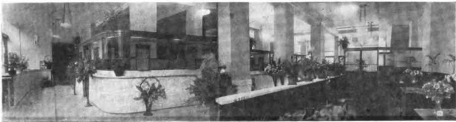
The remodeled and enlarged banking rooms of the Park Trust Co., Worcester, Mass.
