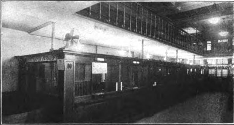
Main Banking Room, New Netherland Bank of New York. "No-Noise" Treatment installed on under side of balcony.
