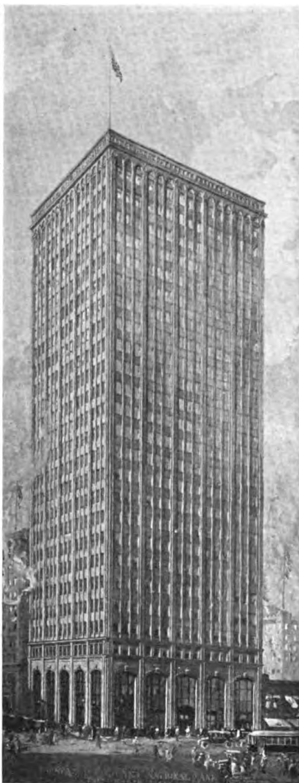
New bank and office building in course of construction for the Farmers and Mechanics National Bank, Fort Worth, Texas. The building will be twenty-six stories, the bank occupying the basement, ground floor and the two mezzanines. The banking room is forty feet high.
