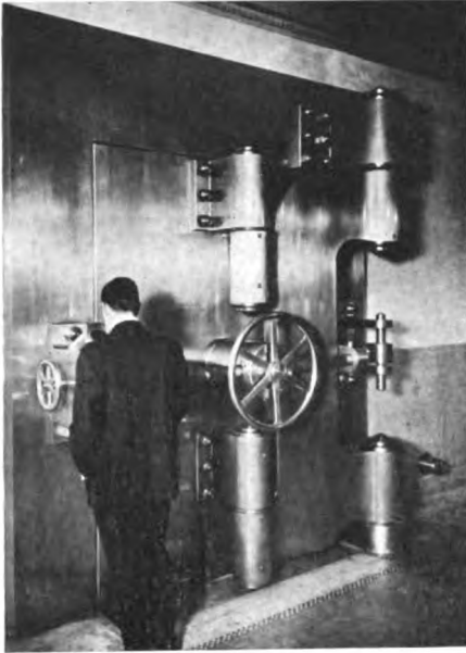
Doors to Safe Deposit Vault, weight about 25 tons
