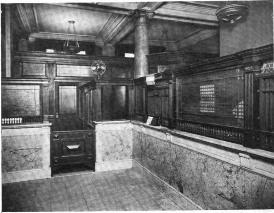
Partial View of Main Banking Room
