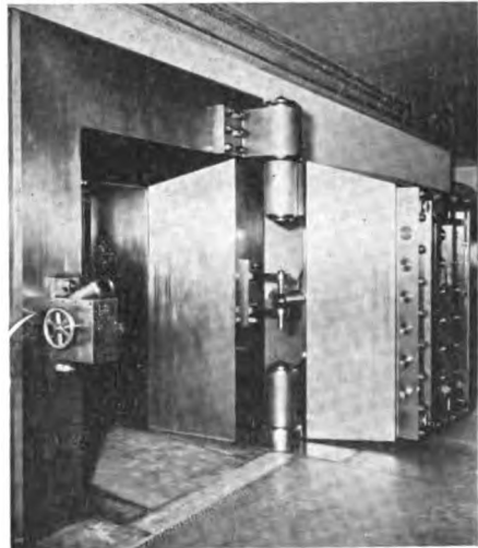
Doors to Safe Deposit Vault open showing extreme thickness
