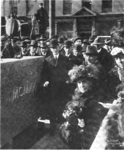
Governor E. I. Edwards is here shown spreading mortar under the corner stone
