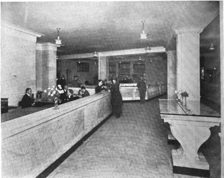
View of Main Banking Room and Officers' Quarters in the Rear
