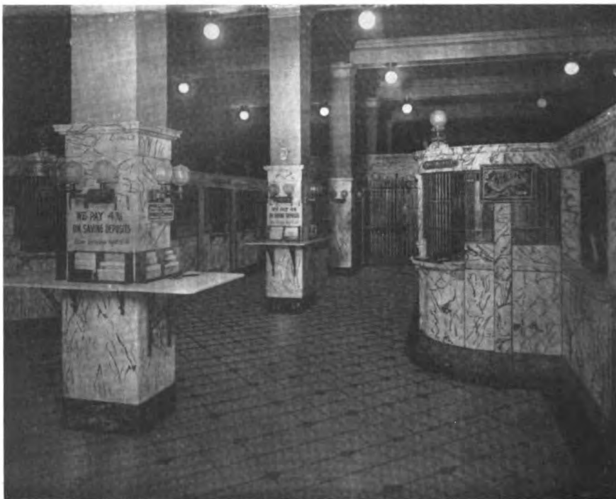
Interior, Cumberland Valley Office, American Trust Company
