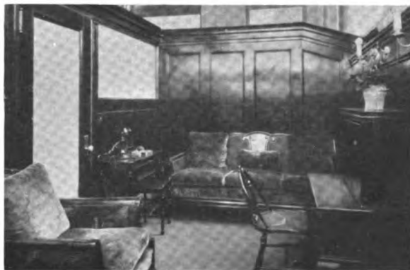
Women's rest room
