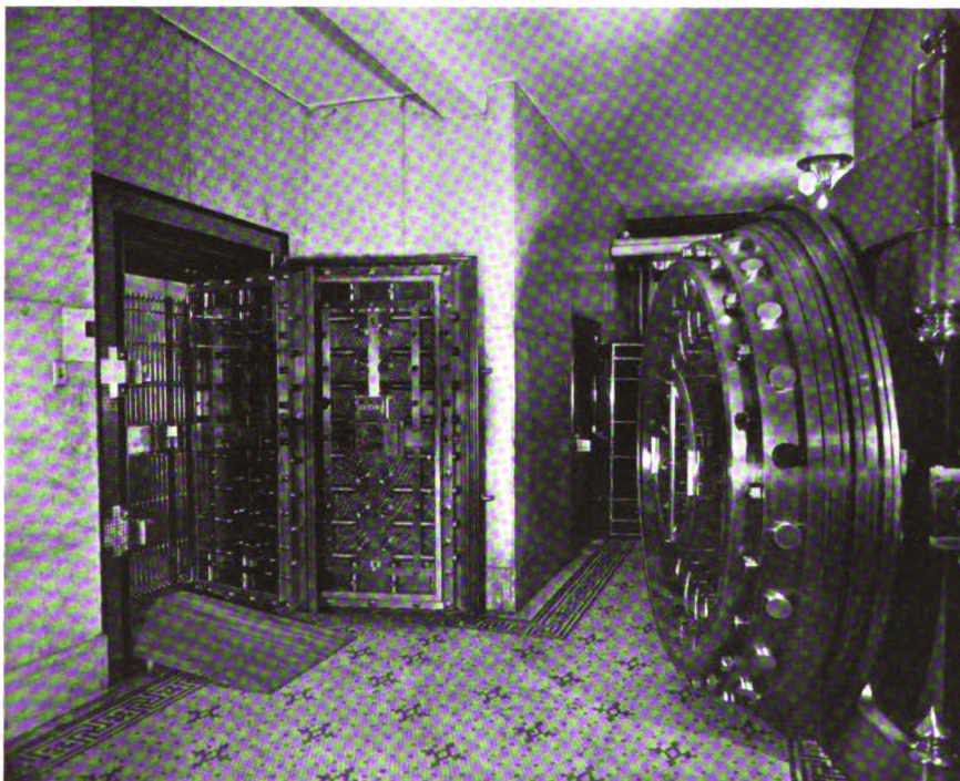
Left to right--Double automatic door, cash vault, fire-proof vault and door to safe deposit vault
