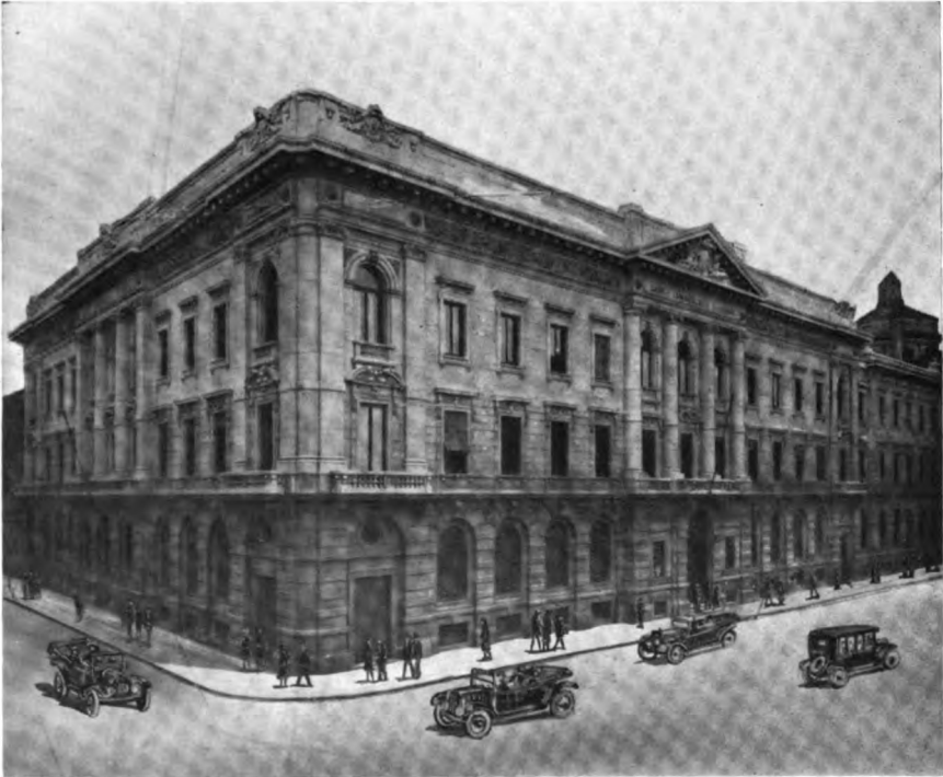
Banca Commerciale Italiana, head office, Milan, Italy
