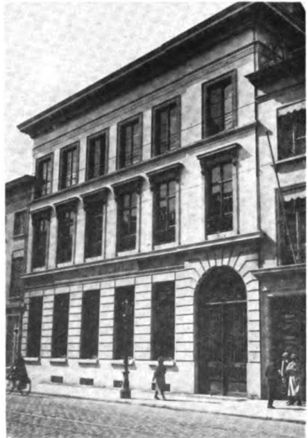
Antwerp office of the Guaranty Trust Company of New York. This new office at 36 Rue de Tanneurs was opened on September 1
