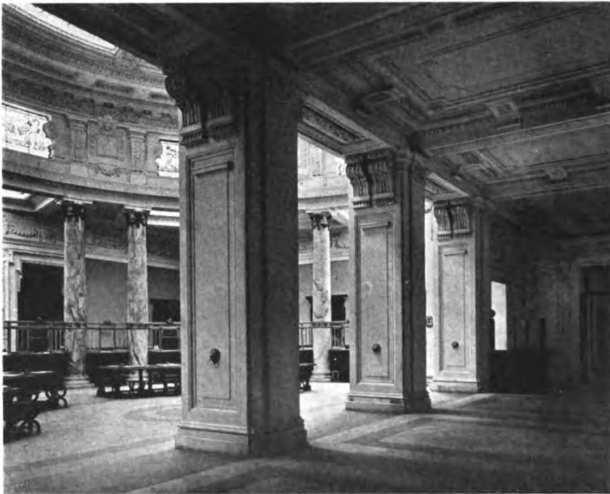
Interior of the Main Banking Room at the Home Office
