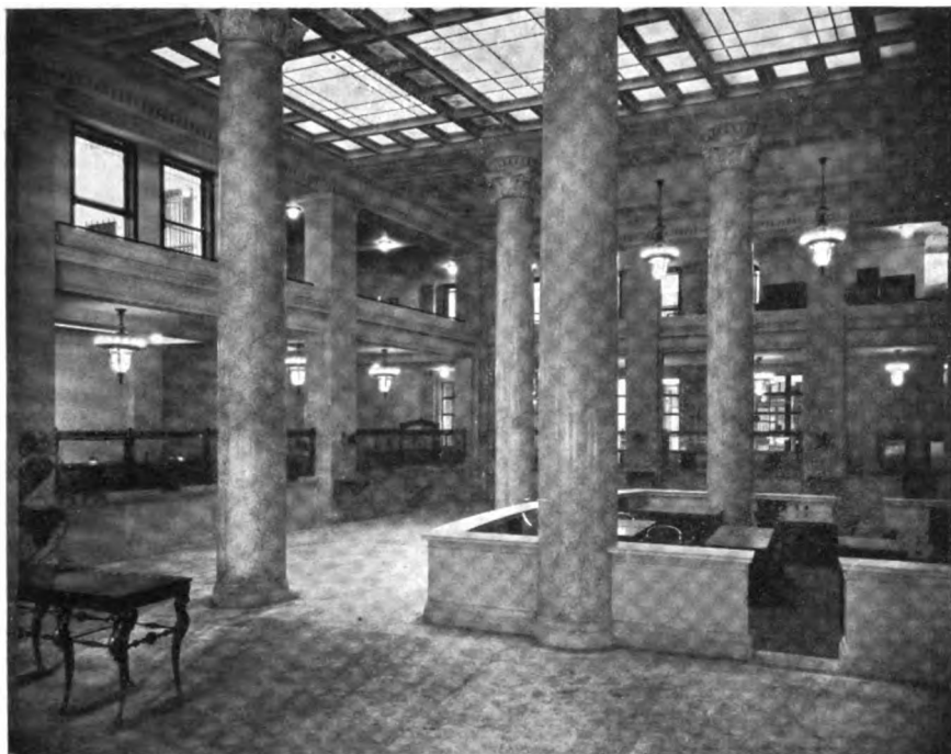
Customers' Lobby and Cashiers' Platform Showing Mezzanine
