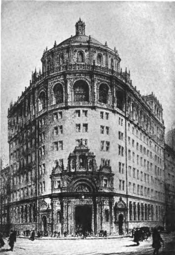
Buenos Aires Branch of the First National Bank of Boston, Mass.
