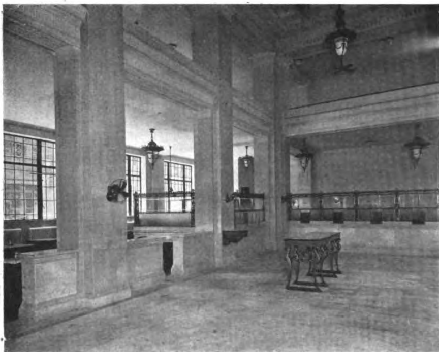
Entrance to Executive Office From Public Lobby
