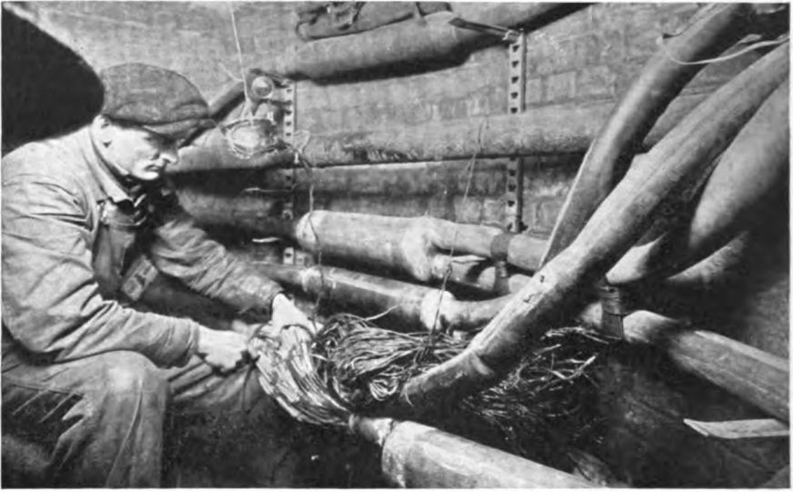
Splicing an underground cable
