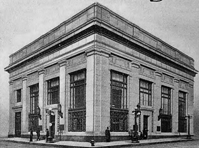
Scott County Savings Bank, Davenport, Iowa. Entire granite super-structure on polished granite base.
