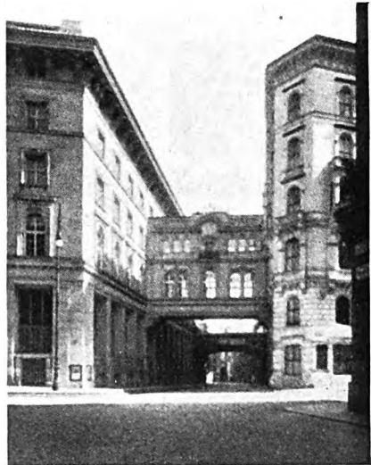
Bridges connecting the new building of the Austrian Society of Credit with the old one
