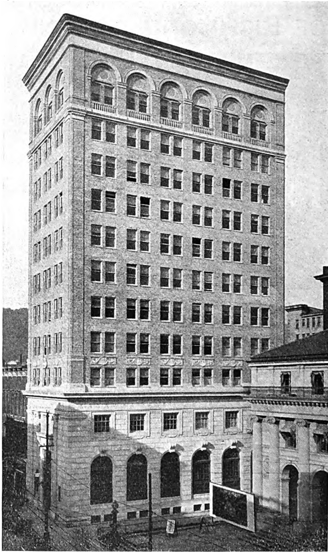
This new building of the Kanawha Banking and Trust Company, Charleston, W. Va., is a twelve story bank and office building, designed in the Florentine Italian Renaissance style. The first two stories above the street are of buff Indiana limestone, the upper stories being of gray brick, very similar to the limestone in color, with terra-cotta trimmings. This building is modern and represents one of the highest types of office building construction. It was planned and supervised by Dennison and Hirons, building specialists, New York
