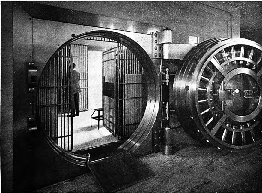
This 18-ton door protects a vault 16 by 16 feet, which houses 2000 safe deposit boxes
