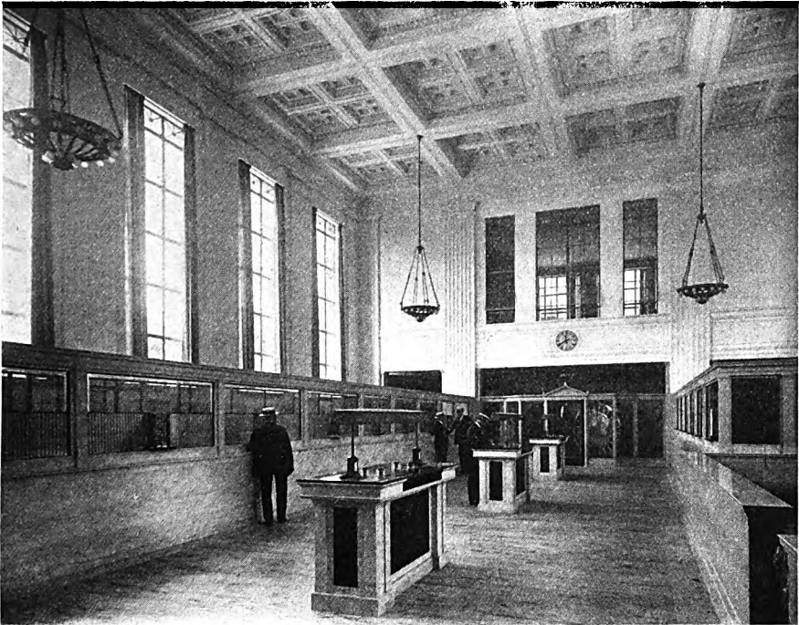
Main banking room looking toward rear, showing entrance to safe deposit vaults
