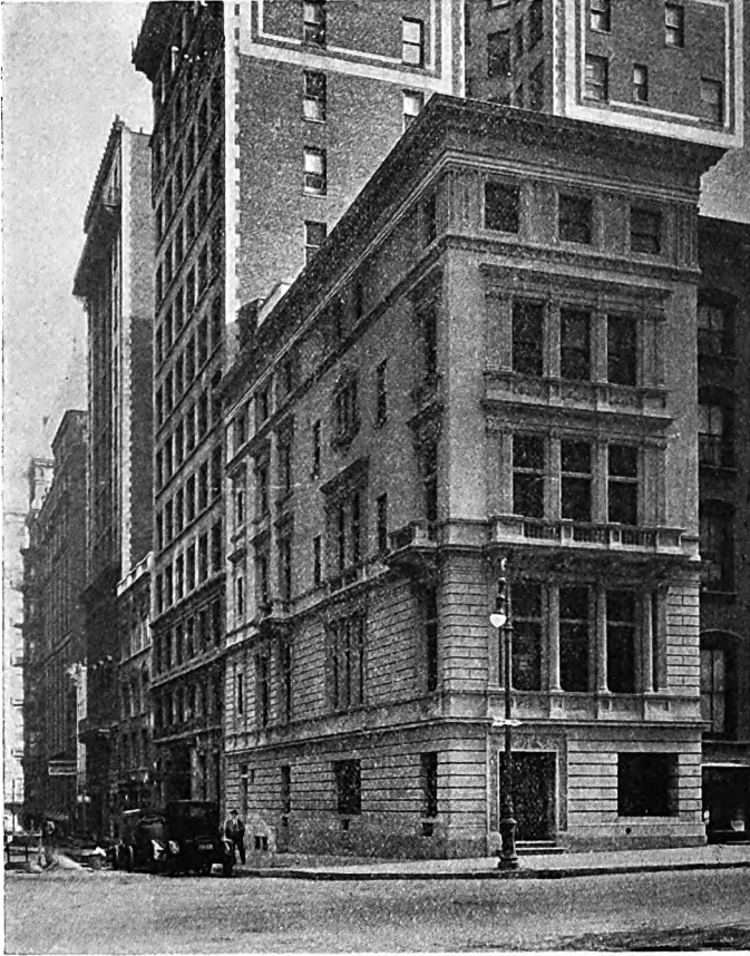
At the southeast corner of Madison avenue and Forty-first street the new midtown office of the American Trust Company and the New York Title and Mortgage Company occupies a prominent site in the city's rapidly developing Grand Central zone
