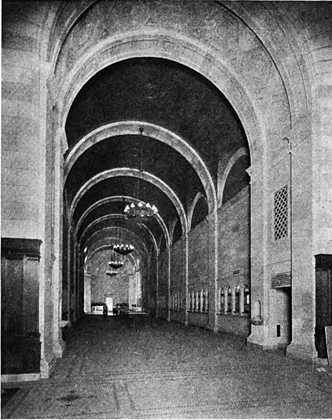
This long arcade, with tellers' wickets on each side, runs from the officers' room to the rear of the building. It is 28 feet wide, a width greater than that of some of Boston's streets, and is three stories high. The vaulted ceiling is of dull gold
