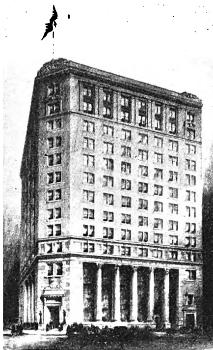
New building for the main office of the Italian Savings Bank at Spring and Lafayette streets, New York. C. P. H. Gilbert of New York was the architect
