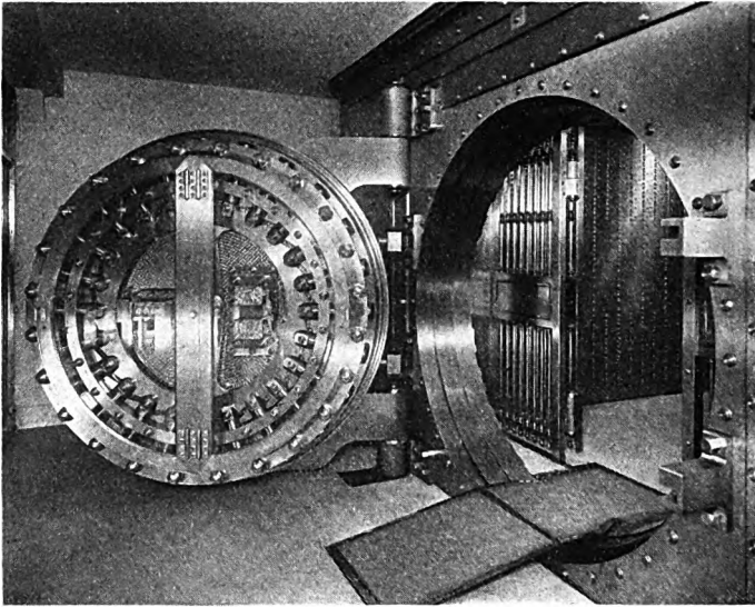
The massive circular door to the vault of the Kajima Bank, Osaka, Japan, is especially constructed to withstand any slight shifting caused by earthquake disturbances. It was built and installed by the York Safe and Lock Company of York, Pa.
