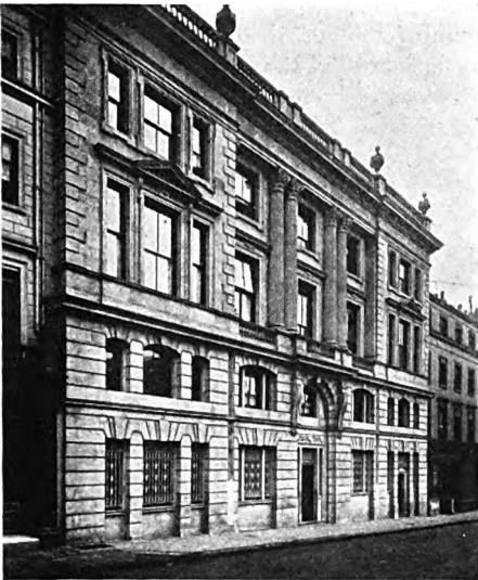
Back of Coutts & Co.'s new building, facing Adelaide street
