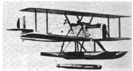
Naval torpedo plane snapped in the act of releasing torpedo
