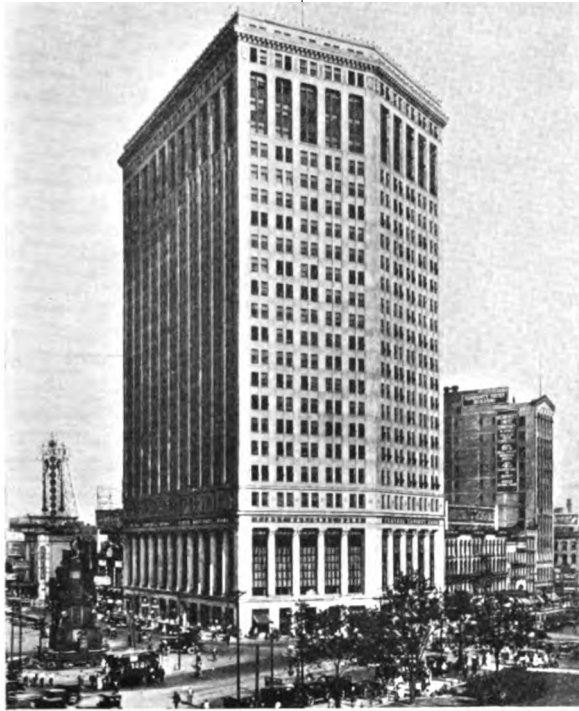
Building of the First National Bank of Detroit, which is equipped with Reed Air Filters
