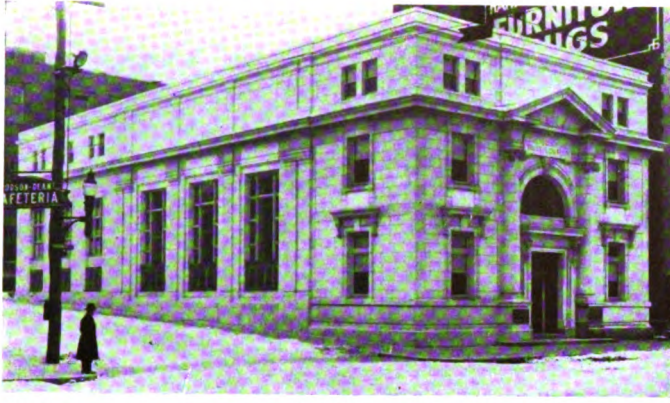
Reconstructed and enlarged building of the Colonial Trust Company, Waterbury, Conn. Alterations were made by the Griswold Building Company, Inc., of New York
