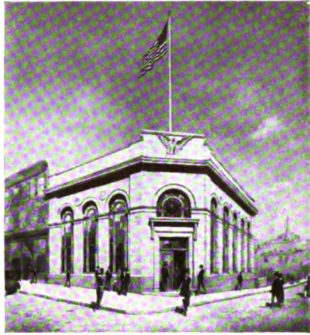
New building of the Union Savings Bank, Mamaroneck, N. Y. This building was planned and erected under the supervision of Morgan, French & Co., Inc., architects and bank engineers, New York.
