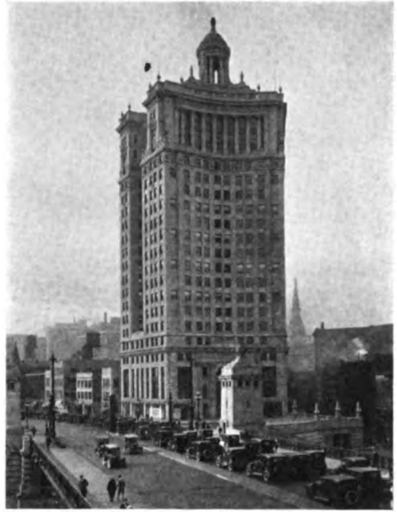
London Guarantee and Accident Insurance Company Building, Chicago. This building was designed and constructed by Dwight P. Robinson & Company, New York
