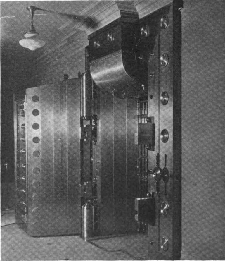
A side entrance to the safe deposit vault, with ventilating duct
