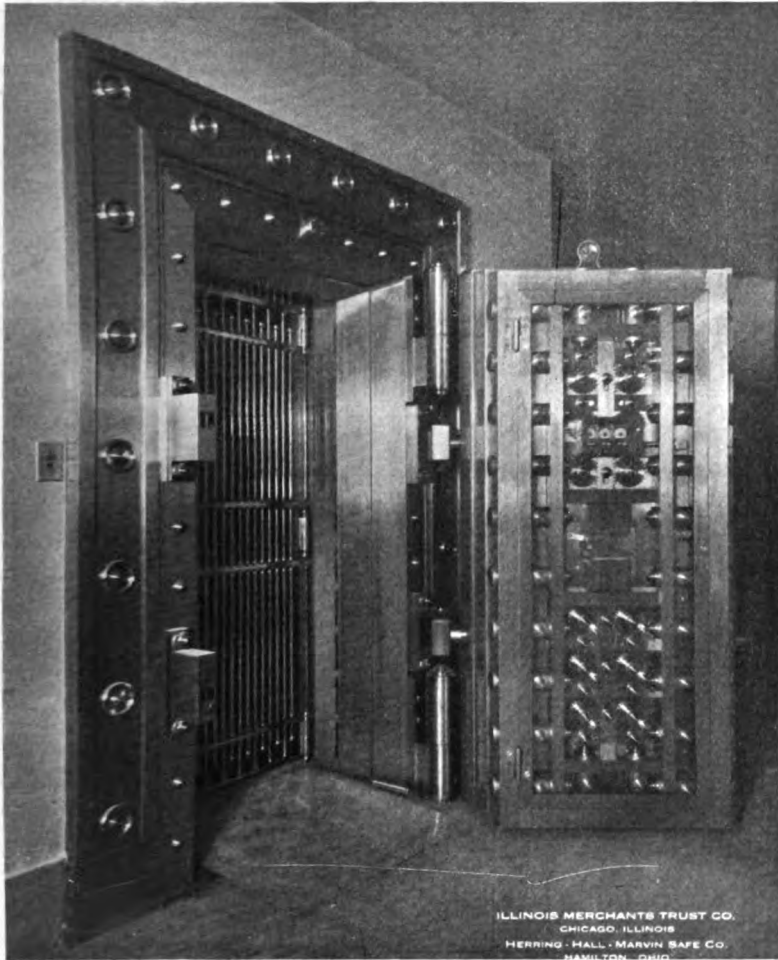
Entrance to trunk vault
