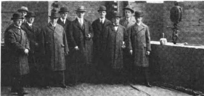
Laying the cornerstone of the new building of the United States Mortgage & Trust Company at Broadway and Seventy-third street, New York. Left to right: W. W. Kelchner, vice-president Charles Diehl, Thornton Earle, Henry Otis Chapman, the architect; Arthur Turnbull and Charles E. Graham, directors; vice-president H. L. Servoss, James Timpson, director; vice-president J. A. Hopper, and president John W. Platten. Mr. Kelchner and Mr. Earle are trustees of the Rutgers Presbyterian Church, which formerly occupied this site
