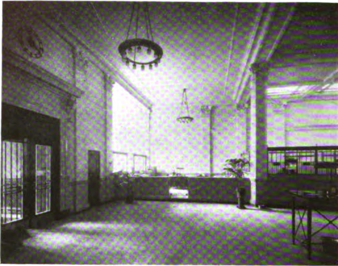
Main Banking Room, Mechanics Bank, Brooklyn, showing Officers' Platform.
