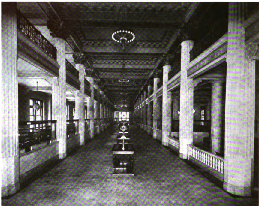
Main lobby, looking from Main street to Fannin street
