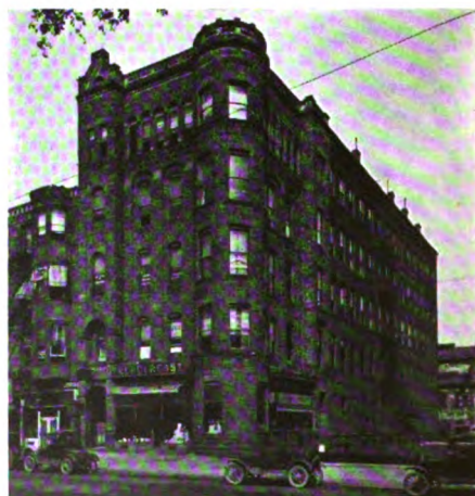
Old building of the Lincoln Trust Company, Scranton' and the new building (to the left) designed by Morgan, French & Co., Inc., architects and bank engineers of New York
