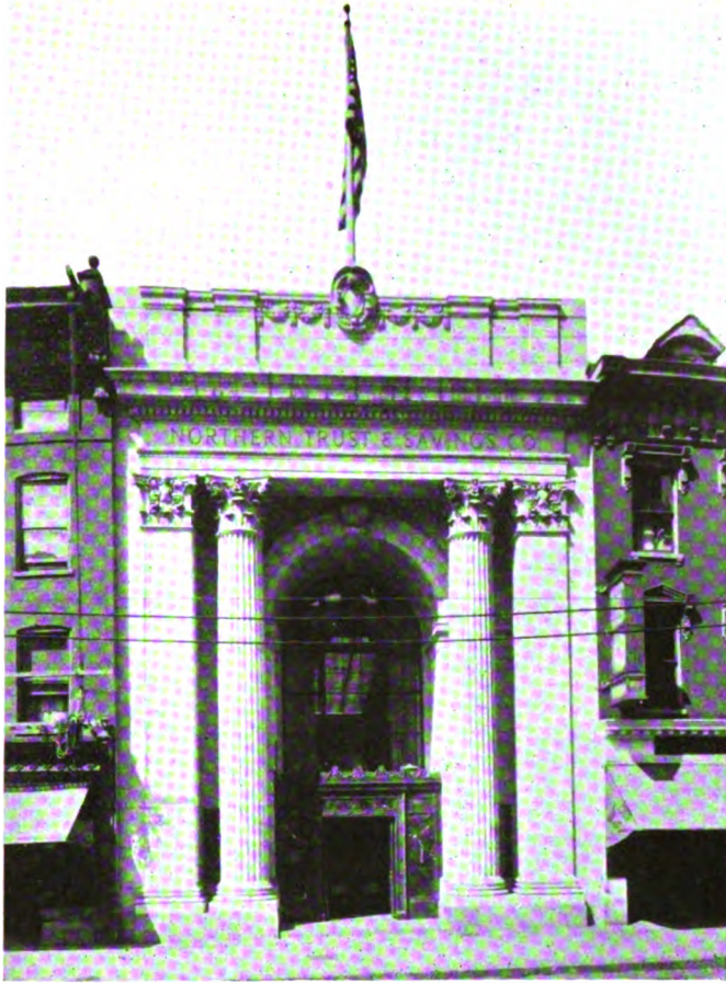
Entrance to new building of Northern Trust and Savings Company, Lancaster, Pa., which was designed, built and equipped by the Griswold Building Company, Inc., New York
