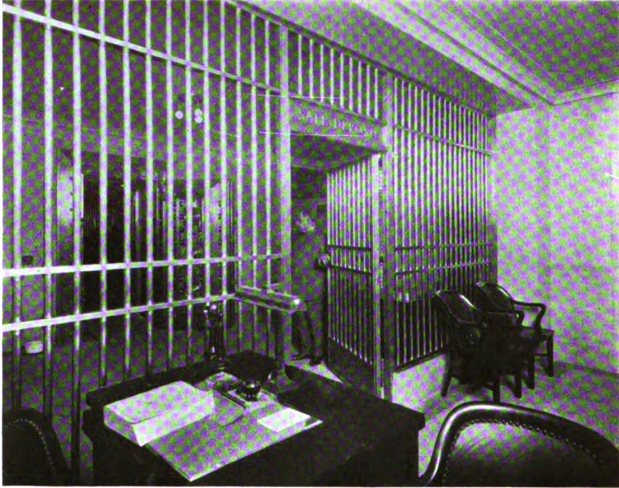
Entrance to safe deposit vaults. All vault work was done by the York Safe and Lock Company of York, Pa.
