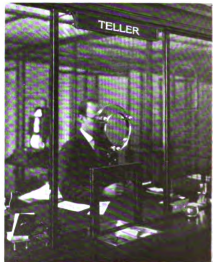
Teller's window, showing how teller is protected against fire-arms
