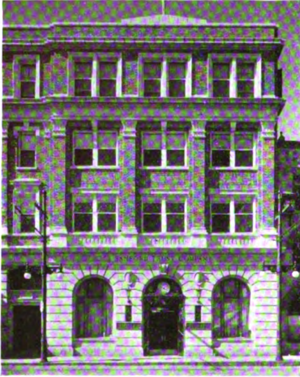
Building of the Sanford Trust Company, Sanford, Maine
