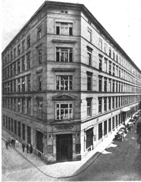
HEAD OFFICE OF THE MERCURBANK
