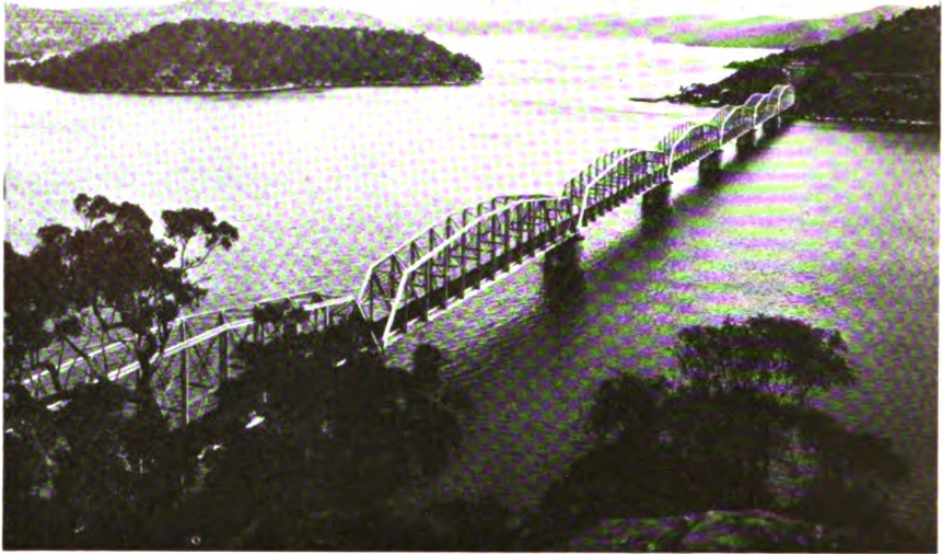
Railway bridge over Hawkesbury river, New South Wales
