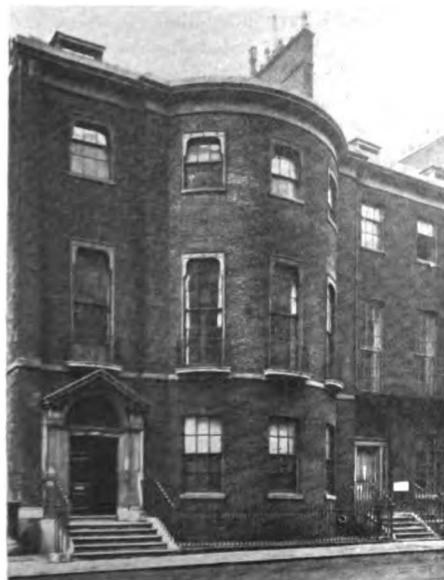
Exterior of 3 Whitehall Place (Holt's Branch) London, S. W. I.
