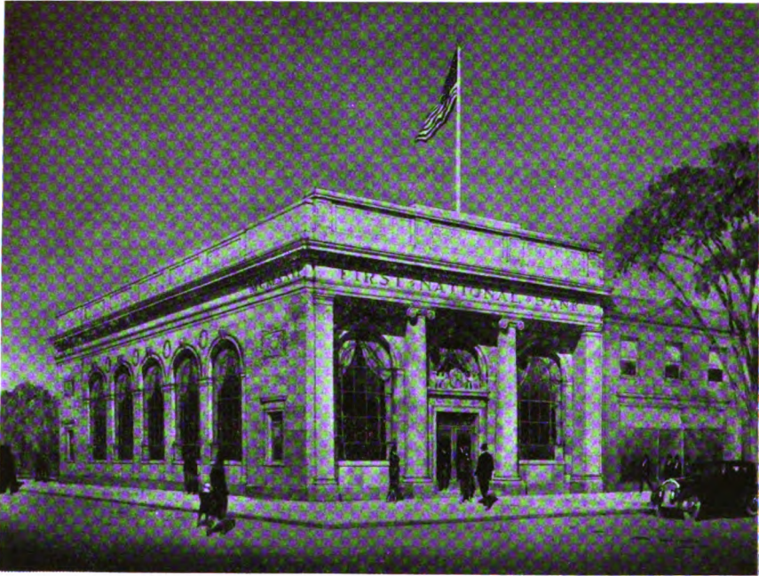
The one story, classical design building of the First National Bank, Ramsey, N. J., designed by Purdy & Davis, architects, New York. The large windows provide plenty of display space for window advertising.
