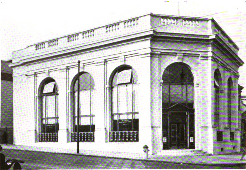
The large windows in the Hibernia Savings and Loan Society's building at San Francisco are equipped with Crittall steel window casements. Bakewell & Brown were the architects.
