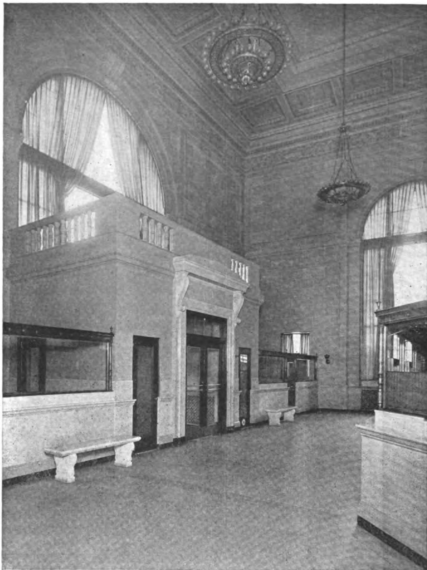
Entrance Lobby, Home Savings Bank, White Plains, N. Y.
