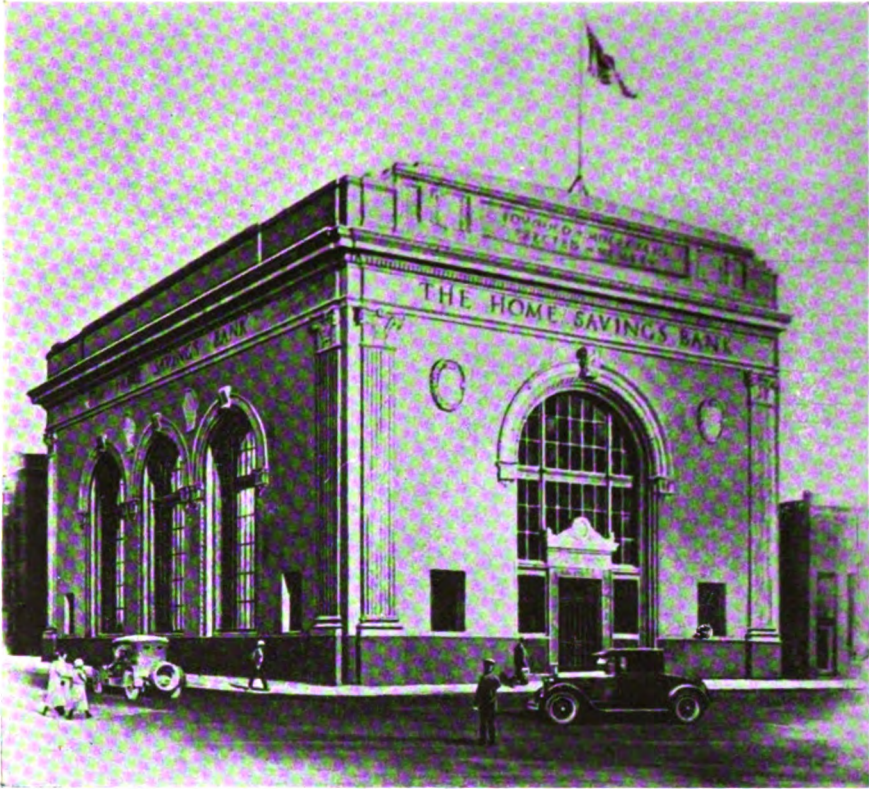
The new building of the Home Savings Bank, White Plains, N. Y., planned and constructed under the supervision of Holmes & Winslow, bank architects, New York. It is individual in character, of Italian Renaissance architecture, faced with variegated Indiana limestone, and is designed to house the bank alone.
