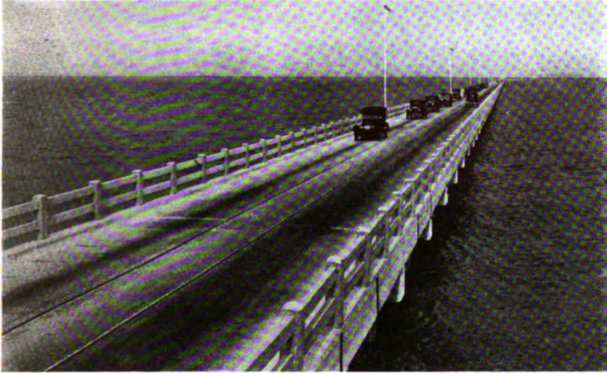
Gandy Bridge, connecting St. Petersburg and Tampa—the longest automobile toll bridge in the world. Built by George S. Gandy of St. Petersburg. In its first year of operation, recently closed, more than 2,000,000 passengers and over 860,000 vehicles crossed the structure
