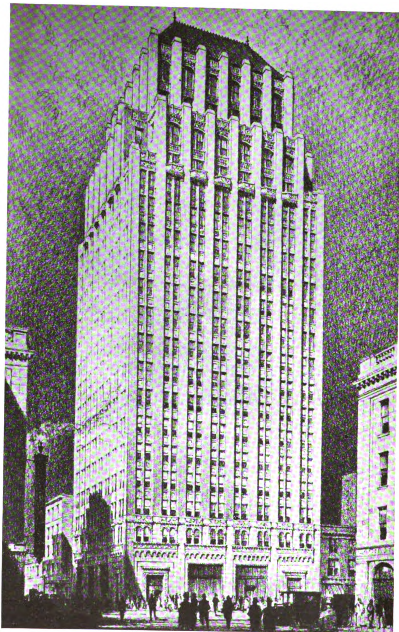
The building of the Fidelity Bank, Houston, Texas, designed with the Mayan motif to express power with a decorative quality, not meticulous ornament
