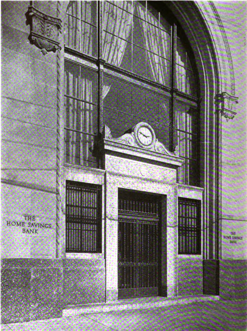
A close-up of the entrance to the Home Savings Bank, White Plains, N. Y., planned and constructed under the supervision of Holmes & Winslow, bank architects, New York. The large arched window over the carved stone doorway with its solid ornamented bronze doors, throws an abundance of light into the main banking room.
