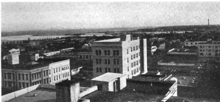
Commercial harbor, St. Petersburg. The city has recently spent $500,000 on dredging the harbor to accommodate ocean going vessels. A new bond issue of more than $1,500,000 for harbor improvements is now under way. The port of St. Petersburg has been a material factor in relieving traffic congestion on freight into Pinellas County.
