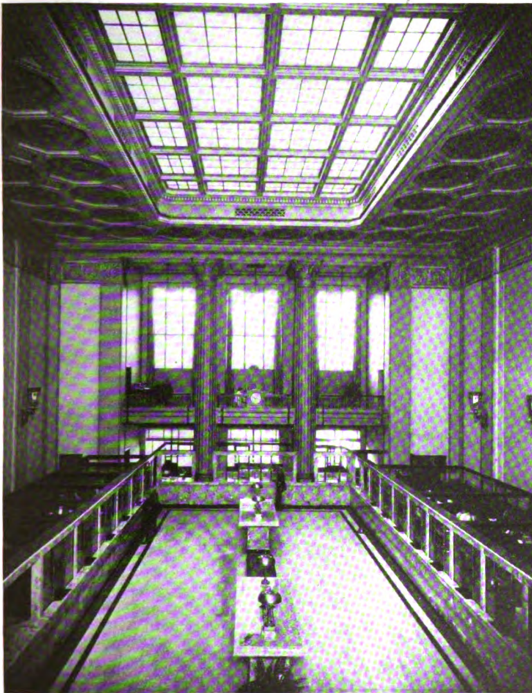
An interior view of the Bank of California, Seattle, Wash. (John Graham, architect) showing the installation of steel window and skylight casements made by the Crittall Casement Window Co., Detroit. The large window and skylight space gives ample light and air to the working quarters in the bank.
