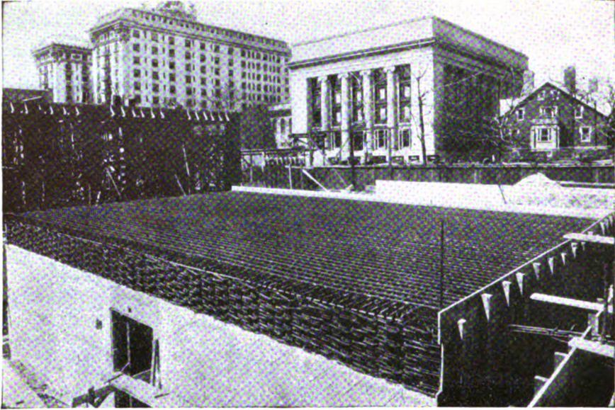
*Rivet-Grip Reinforcement in Top Slab and Walls*
