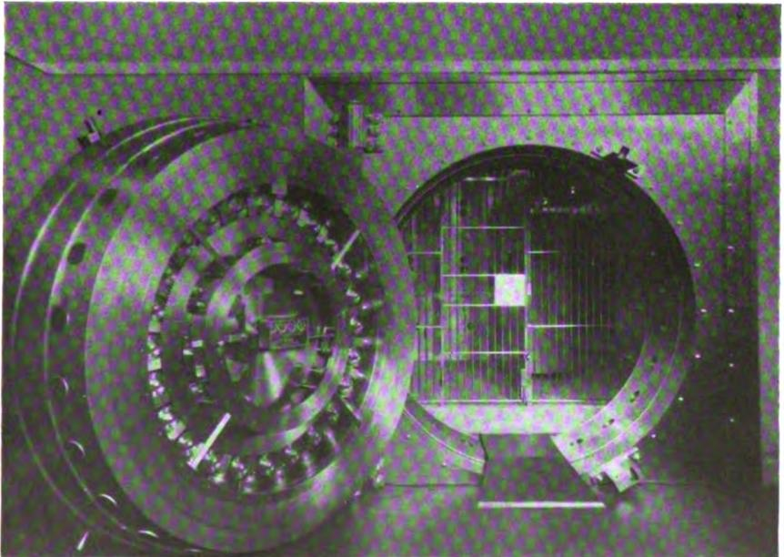
Twenty-six ton door to the safe deposit vault of the Putnam Trust Company, Greenwich, Conn., manufactured and installed by the Herring-Hall-Marvin Safe Co., Hamilton, Ohio, and New York.
