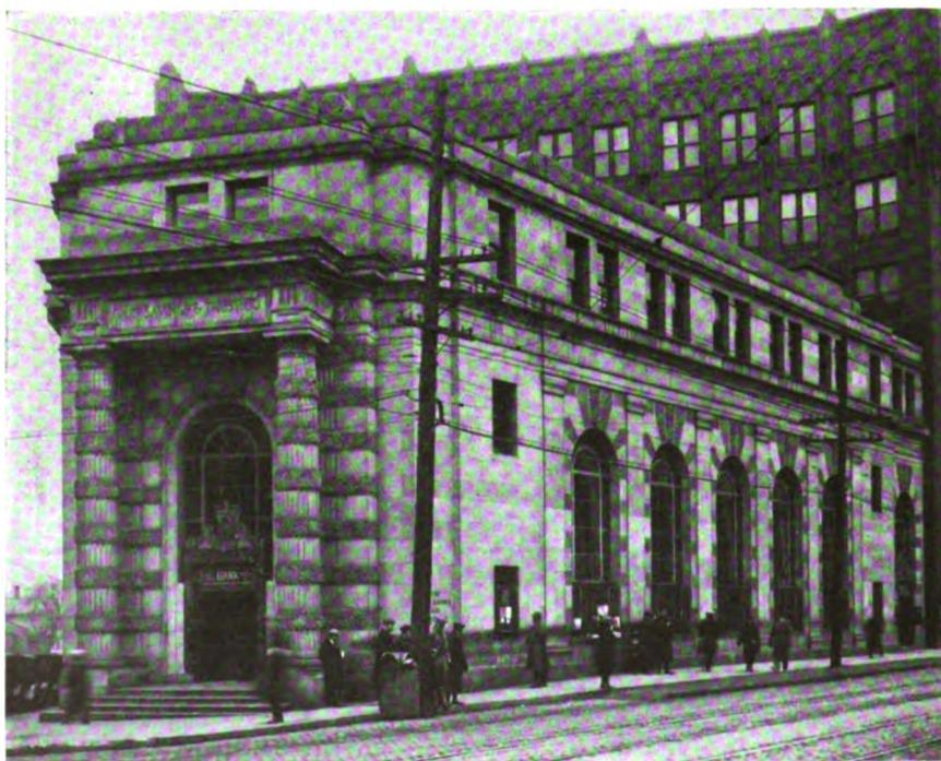
The Ohio Savings and Trust Company, Akron, Ohio, showing the steel window casements installed by the Crittall Casement Window Company, Detroit. Waiker & Weeks were the architects.
