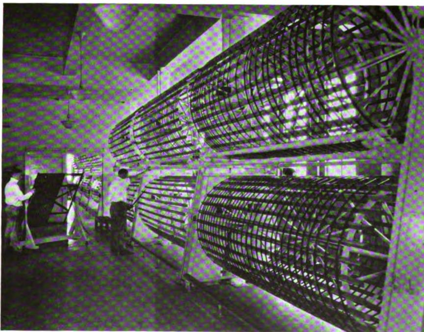
Film drying rooms in a modern film laboratory. The negative drum room is in the foreground and the positive drum room in the background. On these huge drums the developed film is dried by filtered air and made ready for release.
