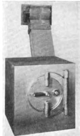
Rotary, Chute and Chest Ready to Install in Building Wall.
