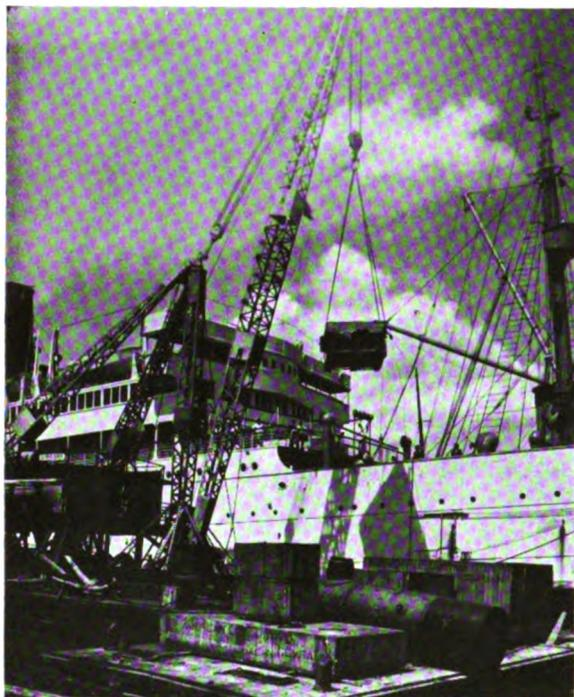
Unloading a twenty-three ton vault door from aboard ship. The transfer and unloading of this huge door as well as other pieces of vault equipment transported on the "S. S. City of Los Angeles," to Honolulu, H. I., was attended without mishap. The shipment included, besides the door, a complete vault installation, one of the most extensive ever shipped abroad. This vault was designed and built by the York Safe and Lock Company of York, Pa., for the Bishop Trust Company of Honolulu.
