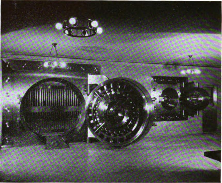
Entrance to the vaults. The vault has two doors, one of thirty tons, the other thirteen, each with four time clocks. The doors lock open as well as closed. Vaults were manufactured and installed by the Herring-Hall-Marvin Safe Company, New York.
