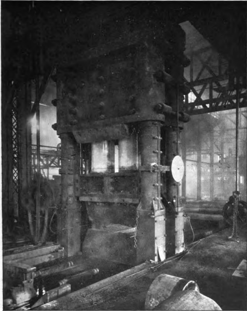
FIG. 5.—Fourteen-thousand Ton Hydraulic Forging Press.
