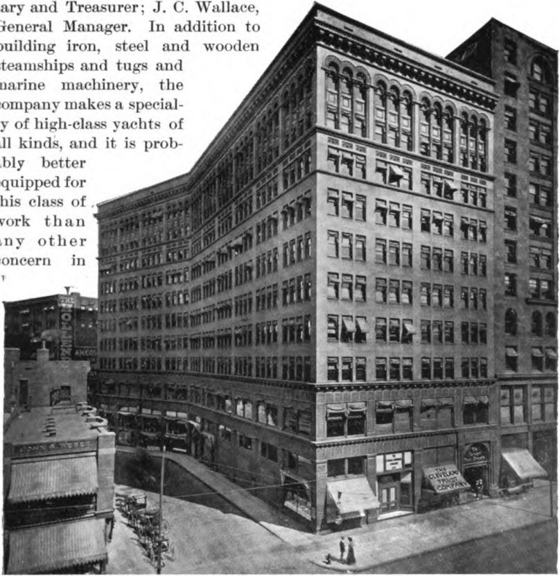
GARFIELD BUILDING—CLEVELAND TRUST COMPANY.
