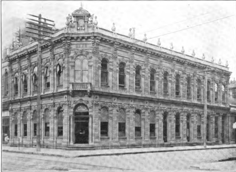
LADD AND TILTON BUILDING.
