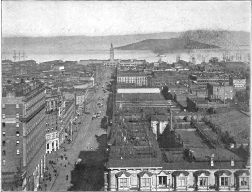
MARKET STREET, LOOKING EAST FROM SPRECKELS BUILDING.
