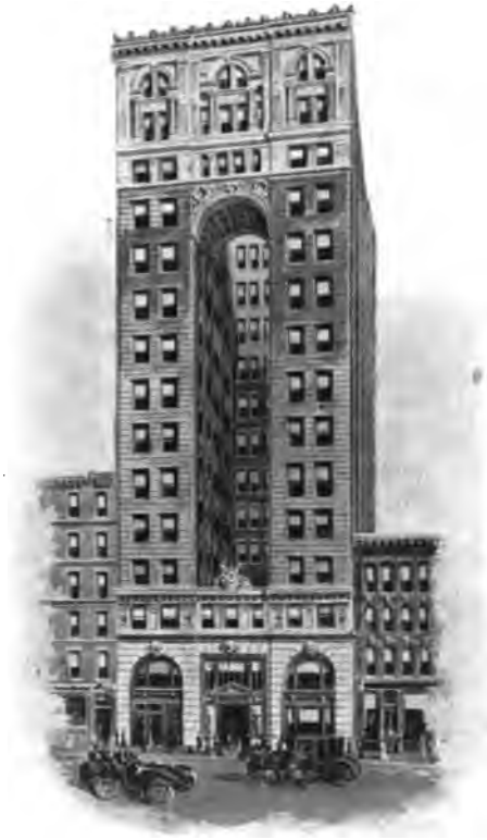
KEYSTONE NATIONAL BANK BUILDING.
