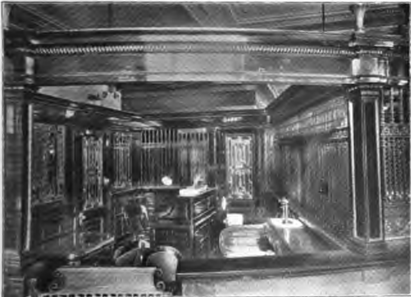
COMMERCIAL NATIONAL BANK, HOUSTON, TEXAS. Glimpse of the Cashier's Office.
