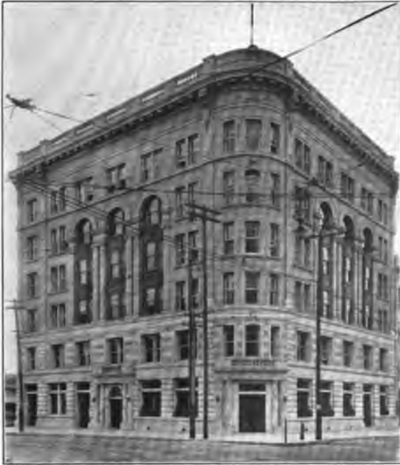
COMMERCIAL NATIONAL BANK BUILDING.
