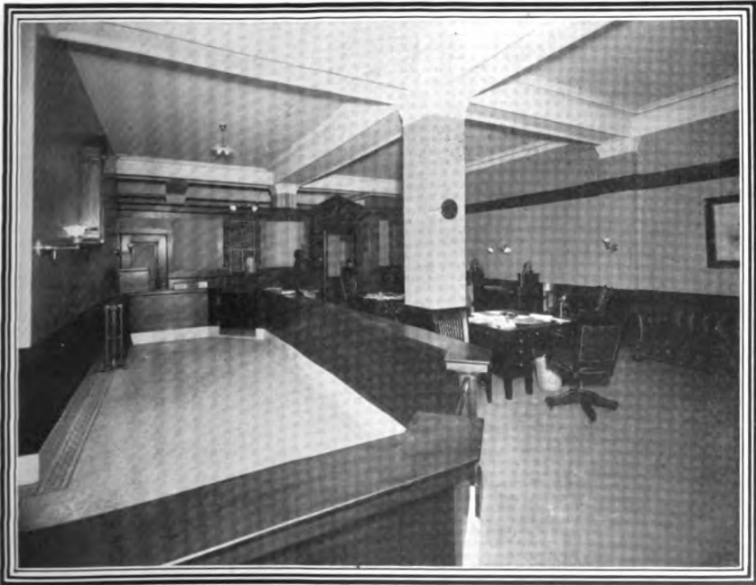
OFFICES OF HARVEY FISK & SONS, BOSTON.
