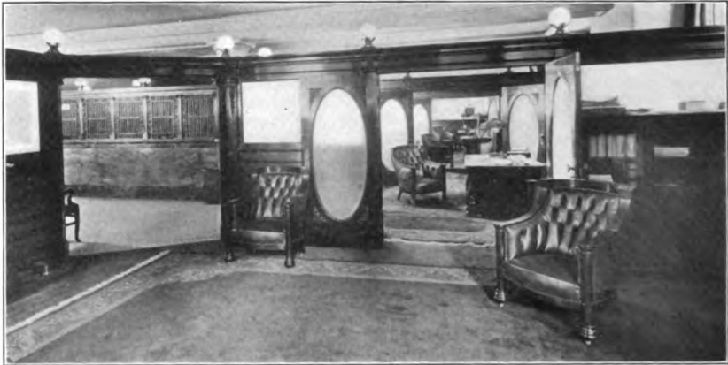
VIEW OF CORRIDOR AND PRIVATE OFFICES OF J. B. RUSSELL & Co., NEW YORK. (Courtesy of Derby Desk Co.)
