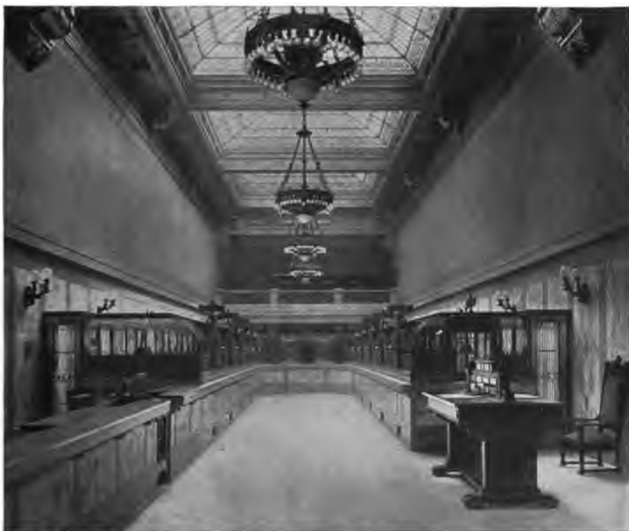
GUARDIAN SAVINGS & TRUST CO., CLEVELAND—THE BANKING ROOM.
