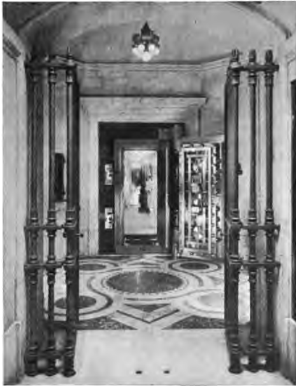
SAFE DEPOSIT VAULTS.
