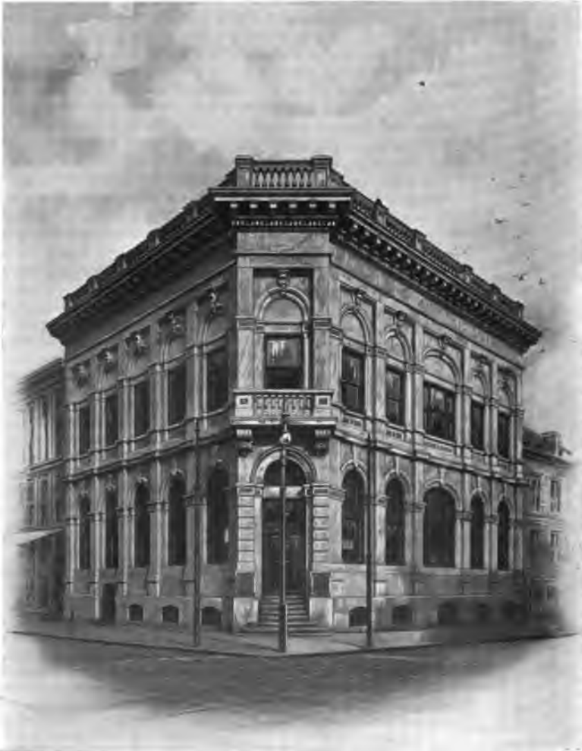
CITIZENS' NATIONAL BANK BUILDING, BALTIMORE.
