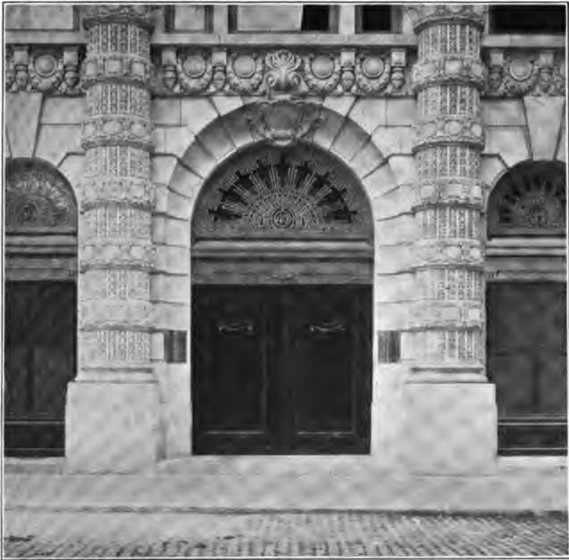
ENTRANCE TO THE ELIOT NATIONAL BANK.
