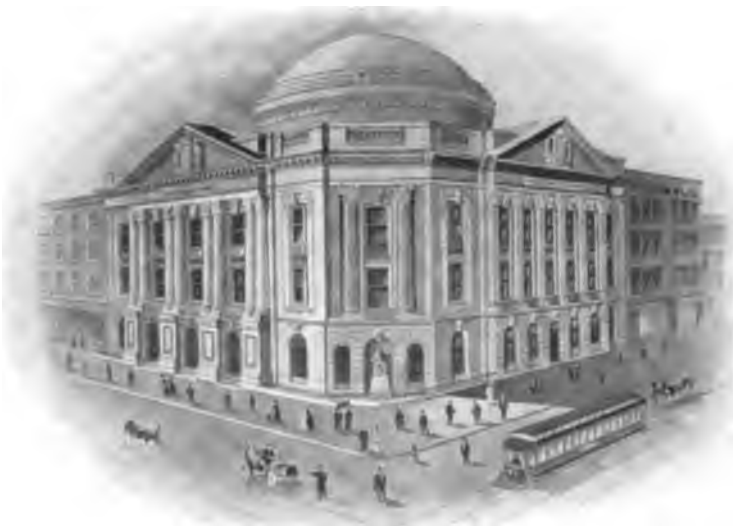
CLEVELAND TRUST CO., CLEVELAND, OHIO. The New Bank Building Now Under Construction.
