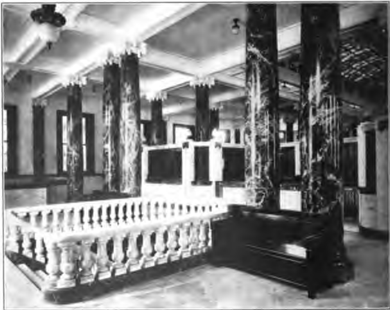
Stairway to Safe Deposit Vaults and Bonds and Securities Department. NATIONAL BANK OF CUBA.
