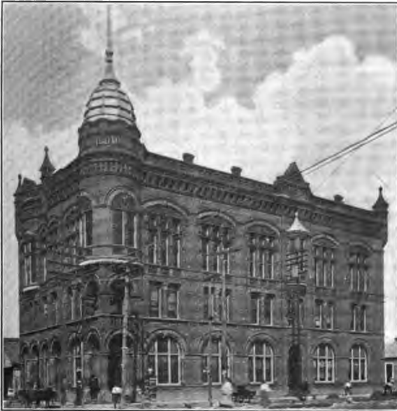
THE BANK'S BUILDING.
