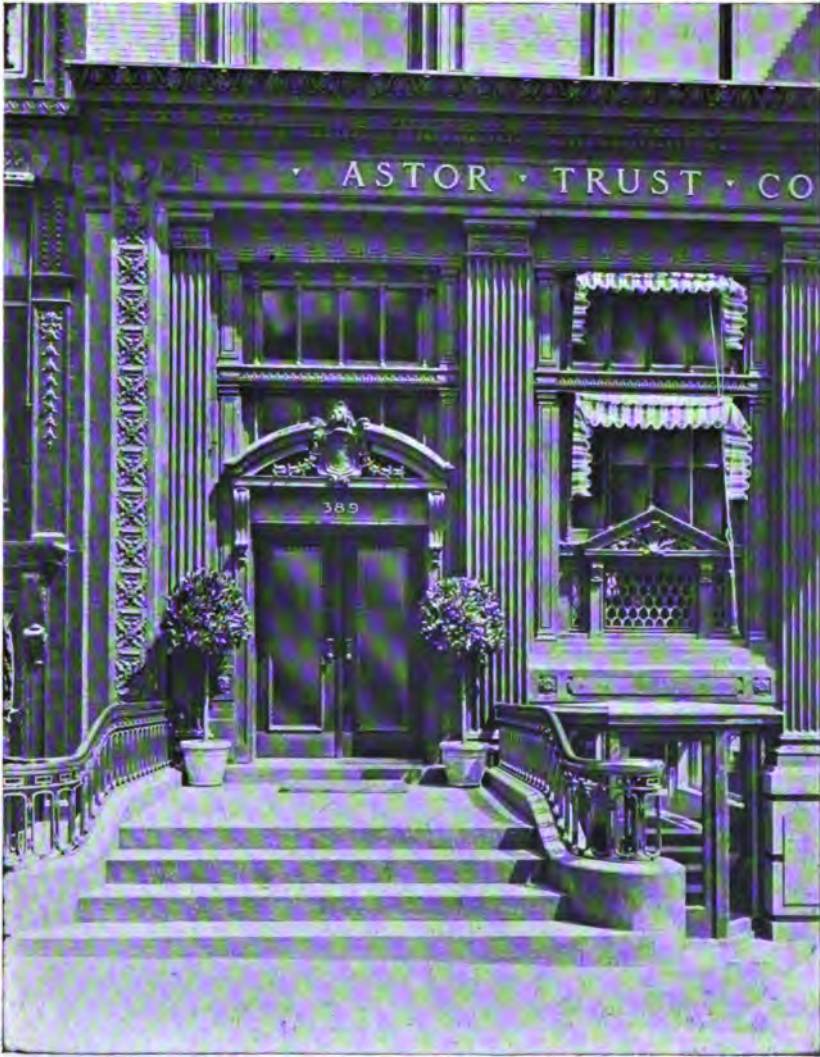
MAIN ENTRANCE, FIFTH AVENUE.
