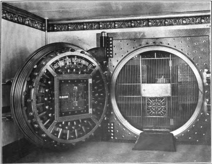
Massive Door and Vault.
