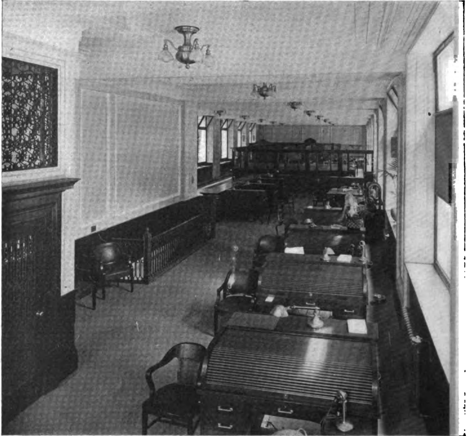
Main Banking Room.
