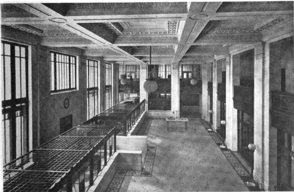
Banking Room from Mezzanine Floor.
