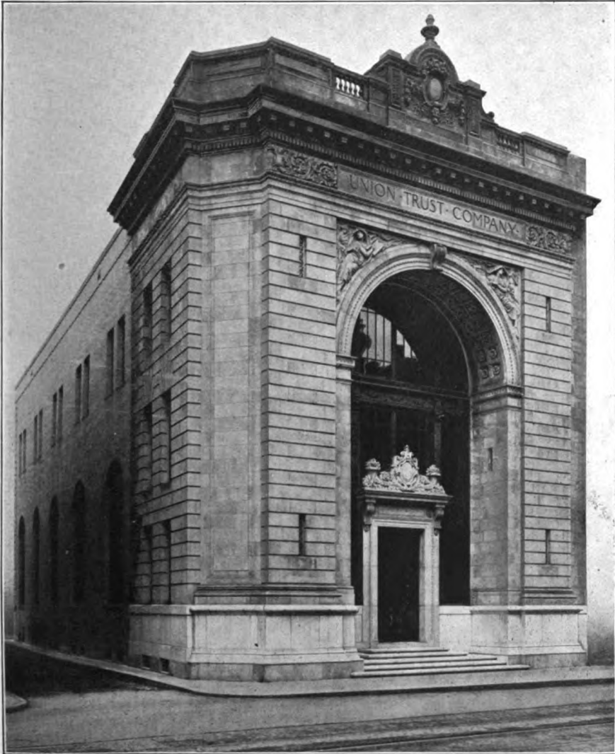
The New Banking House of the Union Trust Company, Springfield, Mass.
