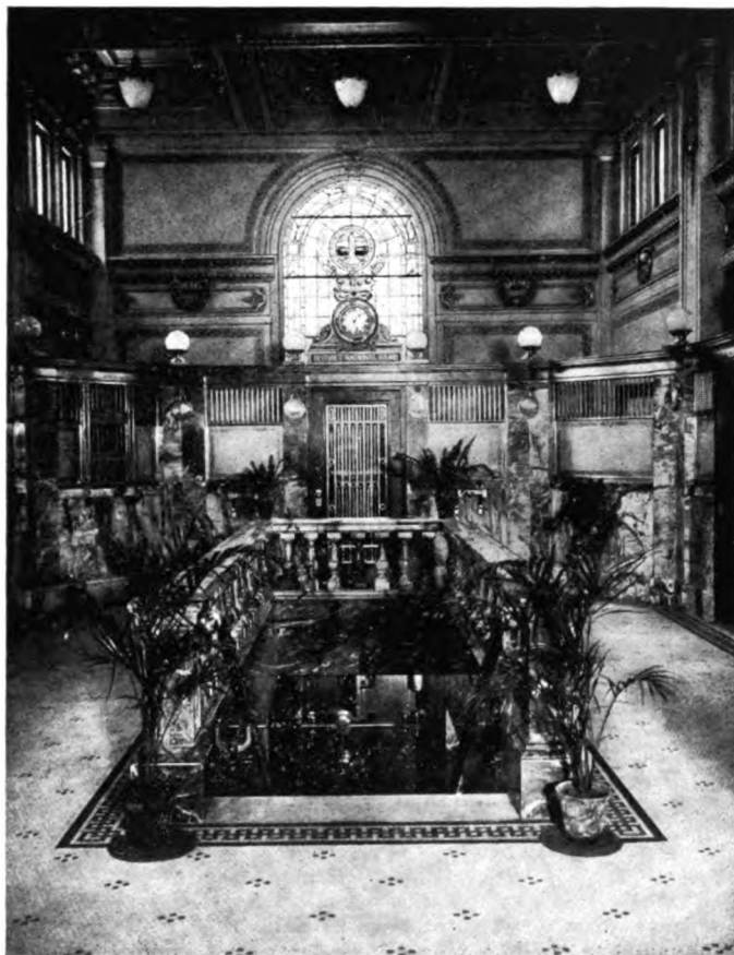
GRAND MARBLE STAIRWAY
