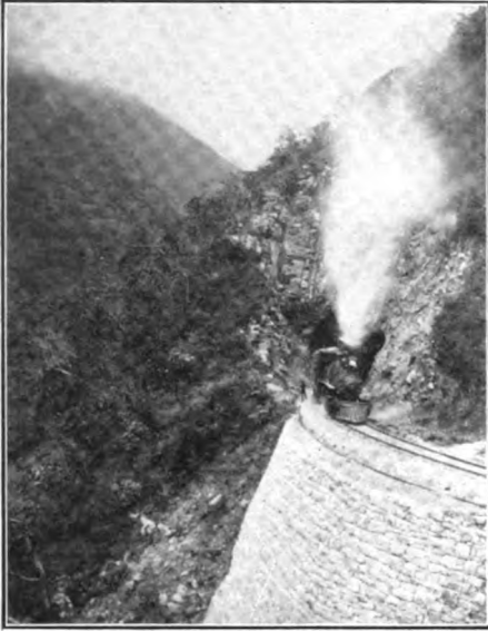
TUNNEL NO. 5—TAMASOPO CANYON IN PICTURESQUE MEXICO
