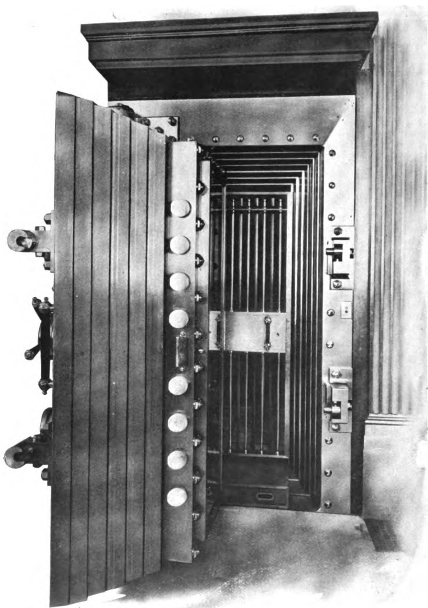
A TYPICAL MODERN SINGLE DOOR OF COMPOSITE CONSTRUCTION, EIGHTEEN INCHES THICK
