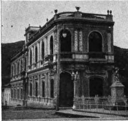
AMERICAN LEGATION BUILDING—BANK BELOW— IN TEGUCIGALPA, HONDURAS
