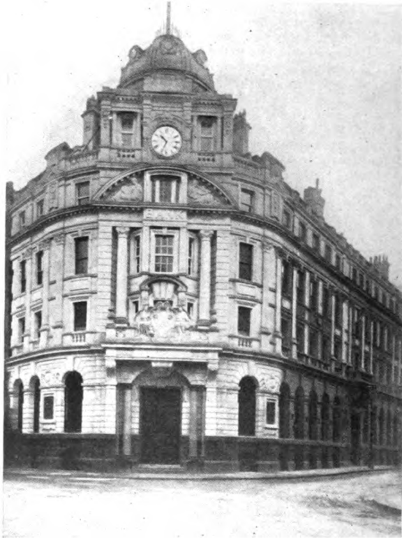
LONDON AND SOUTHWESTERN BANK, LTD. HEAD OFFICE
