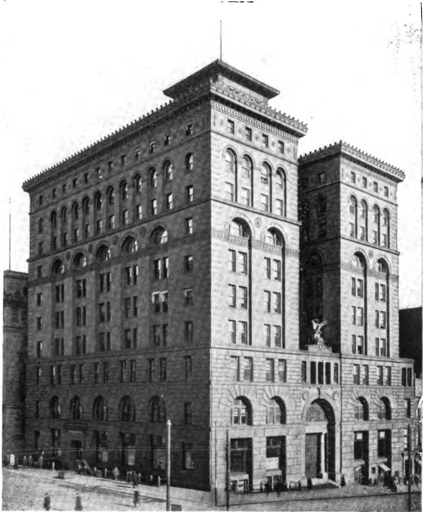
OMAHA NATIONAL BANK BUILDING, SEVENTEENTH AND FARNUM STREETS, OMAHA, NEB.
