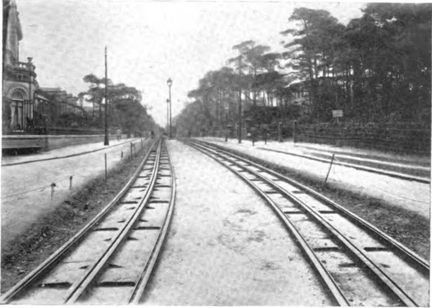
TRACK-CONSTRUCTION WORK IN BOURNEMOUTH, ENGLAND
