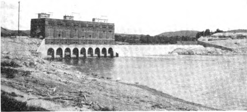
HYDRO-ELECTRIC POWER-HOUSE ON THE CONNECTICUT RIVER
