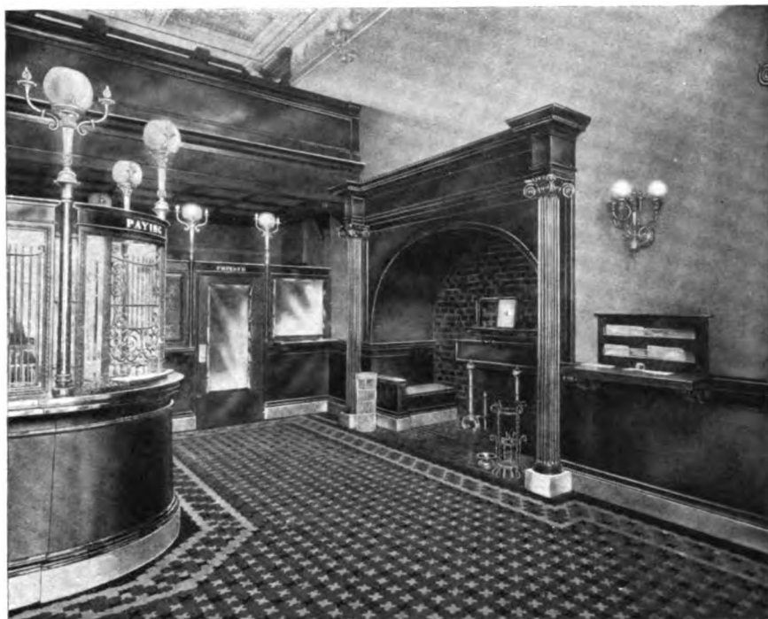
INTERLOCKING RUBBER TILING AS LAID IN THE COUNTY SAVINGS BANK AND TRUST COMPANY OF SCRANTON, PA.
