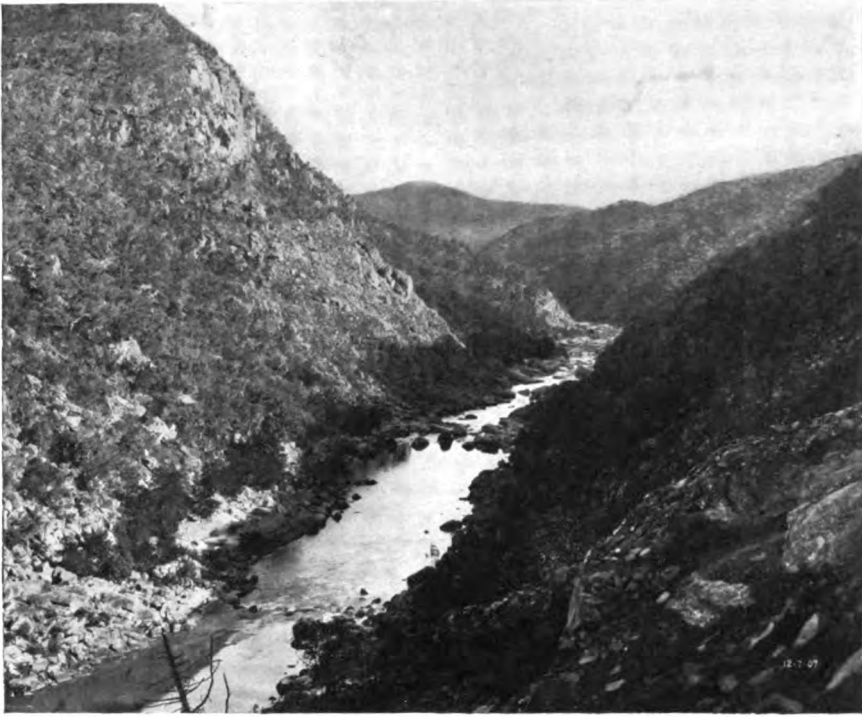
BARREN JACK DAM SITE, FROM TRAM ROAD. THIS IS THE GORGE ACROSS WHICH A DAM TWO HUNDRED FEET HIGH IS BEING BUILT, TO IMPOUND 33,000 MILLION CUBIC FEET OF WATER
