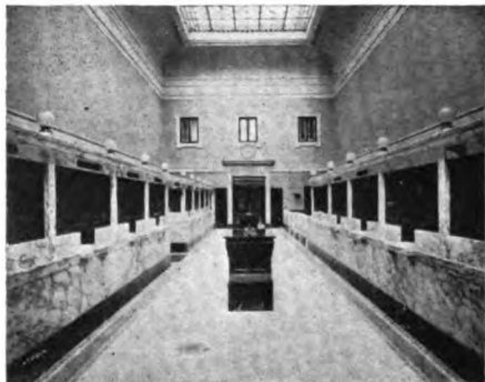
LOOKING TOWARD MAIN ENTRANCE
