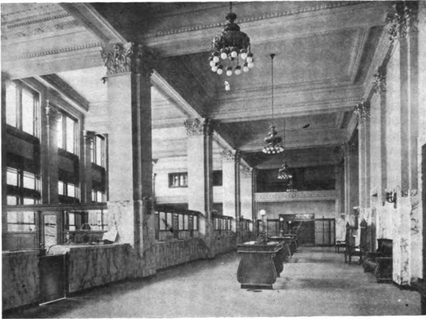
VIEW OF LOBBY, SHOWING A CORNER OF THE OFFICERS' QUARTERS, TELLERS' WINDOWS IN COMMERCIAL DEPARTMENT, SAFE DEPOSIT VAULT AND MEZZANINE FLOOR IN REAR
