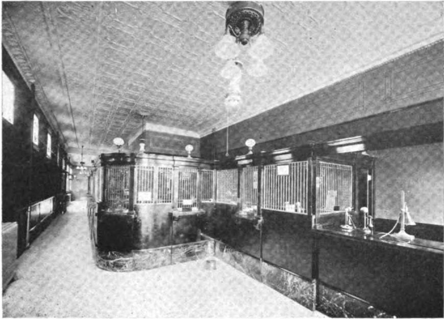
MAIN LOBBY, UNION BANK & TRUST CO., JACKSON, TENN.
