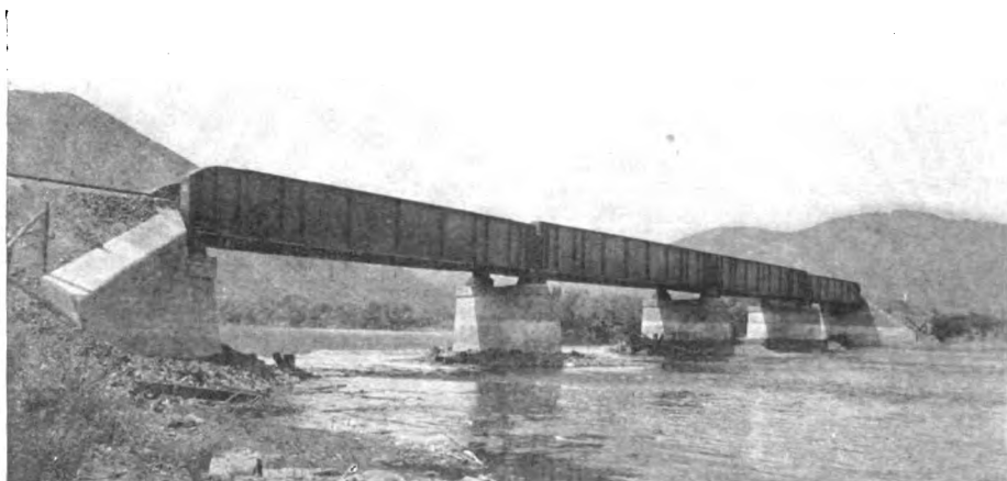
BRIDGE 13 OVER THE JEFFERSON RIVER, BUTTE LINE
