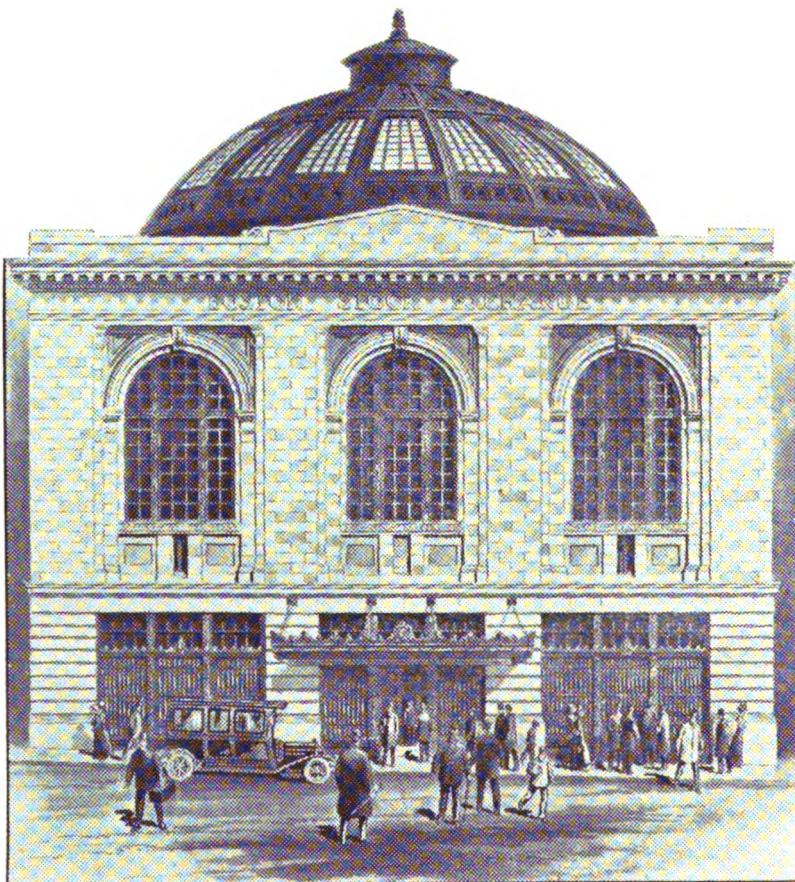
CONGRESS STREET OFFICE COMMONWEALTH TRUST COMPANY, IN NEW BOSTON STOCK EXCHANGE BUILDING
