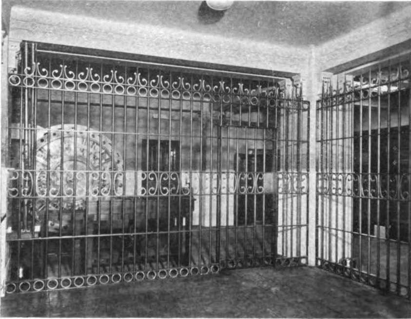
SAFE DEPOSIT VAULTS, AMERICAN NATIONAL BANK, SAN DIEGO, CAL.
