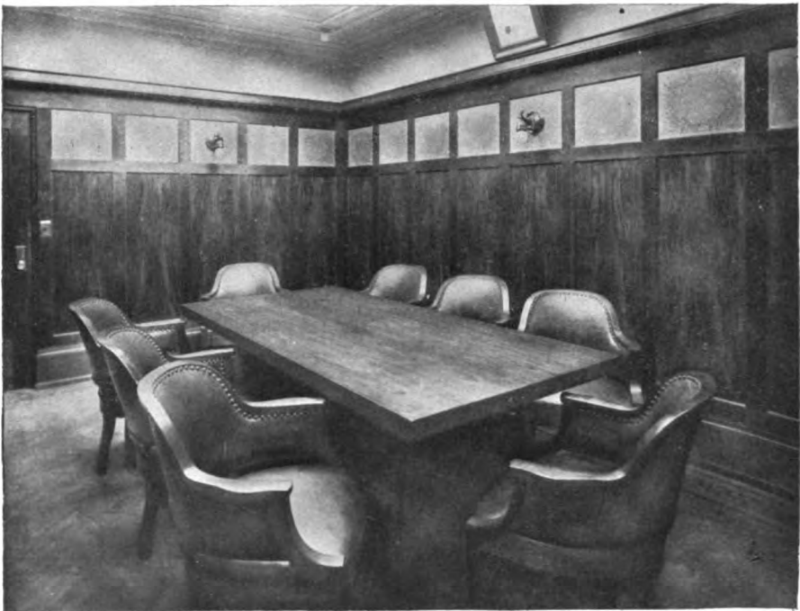
DIRECTORS' ROOM, AMERICAN NATIONAL BANK, SAN DIEGO, CAL.
