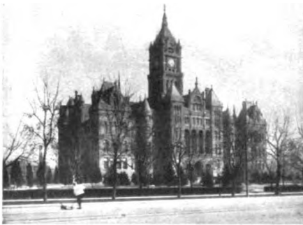
CITY AND COUNTY BUILDING, SALT LAKE CITY; COST A MILLION AND WORTH IT
