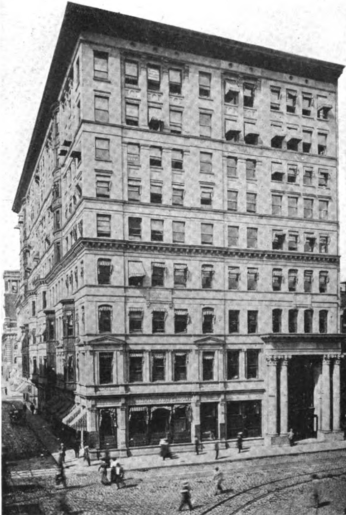
REMODELED BUILDING OF THE INDUSTRIAL TRUST CO., PROVIDENCE, R. I.
