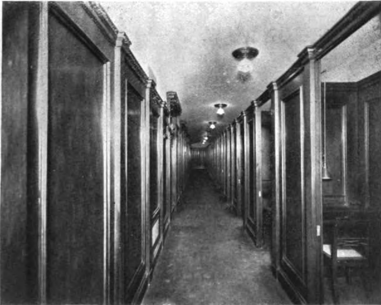
CORRIDOR SHOWING ARRANGEMENT OF SMALL COUPON ROOMS, FIRST NATIONAL SAFE DEPOSIT VAULTS
