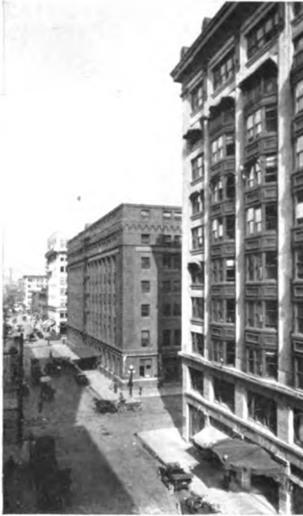
OAK STREET, LOOKING WEST FROM FOURTH STREET, PORTLAND, OREGON
