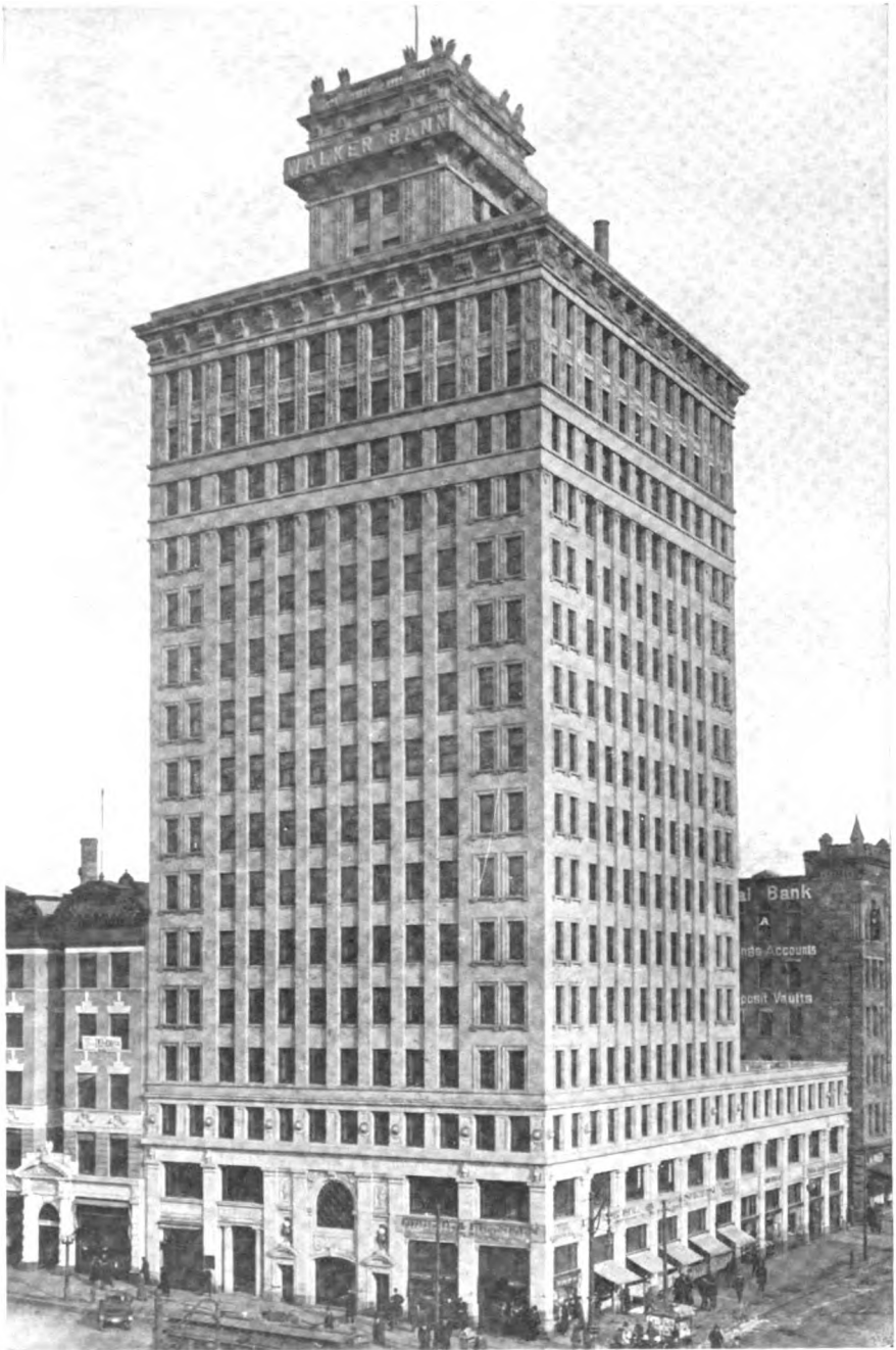
WALKER BROTHERS BANK BUILDING, SALT LAKE CITY
