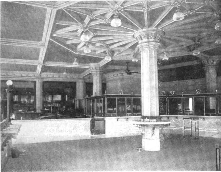
PORTION OF PUBLIC SPACE, MAIN LOBBY, LOWRY NATIONAL BANK, ATLANTA, GA.
