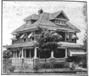
Residence of Mrs. Kirchner, Lanerth, Pa. Covered with J-M Transite Asbestos Shingles.
