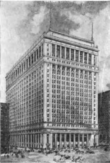
NEW BUILDING BEING ERRECTED FOR THE CONTINENTAL AND COMMERCIAL NATIONAL BANK, CHICAGO, ILL.
