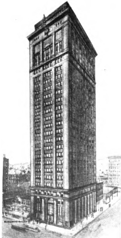
NEW TWENTY-FIVE STORY BUILDING BEING ERECTED FOR THE JEFFERSON COUNTY SAVINGS BANK, BIRMINGHAM, ALA.
