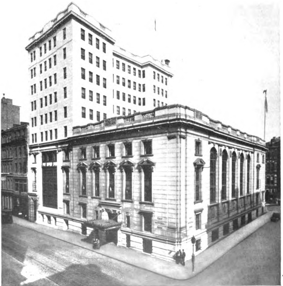
RECENTLY COMPLETED ADDITION TO THE FIRST NATIONAL BANK BUILDING, BOSTON
