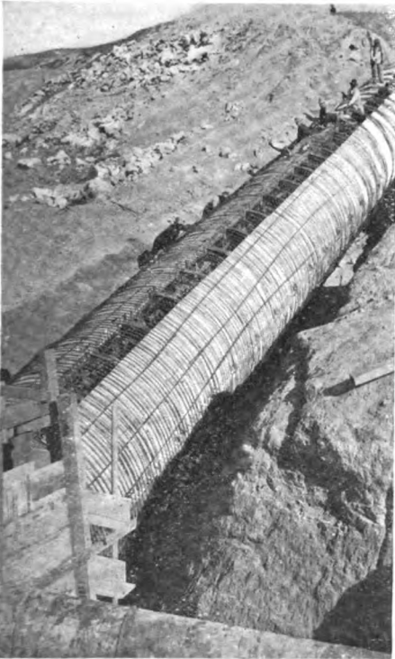
BUILDING THE ELSMERE CONCRETE SIPHON
