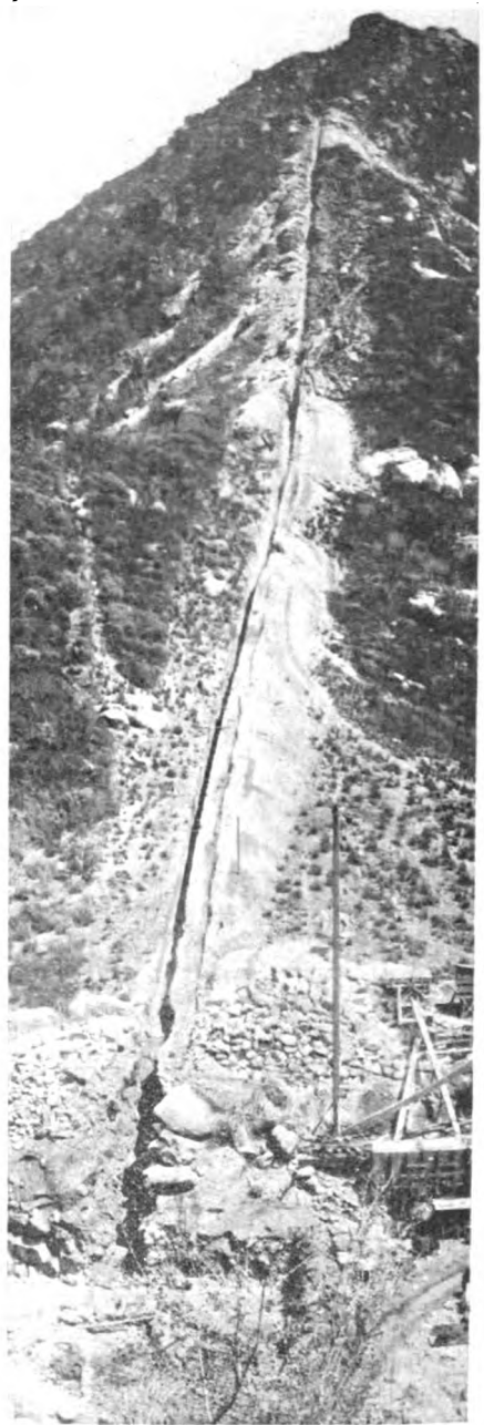
EXCAVATION FOR THE PENSTOCK FROM THE TOP OF PIPE LINE HILL TO THE POWER-HOUSE SITE AT BASE OF THE MOUNTAIN
