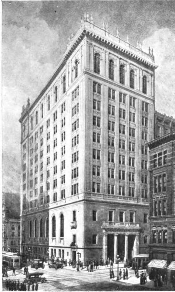
THE DOMINION BANK OF CANADA—NEW HEAD OFFICE BUILDING IN COURSE OF CONSTRUCTION, TORONTO
