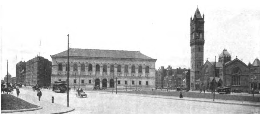
COPLEY SQUARE—THE PUBLIC LIBRARY AND NEW OLD SOUTH CHURCH
