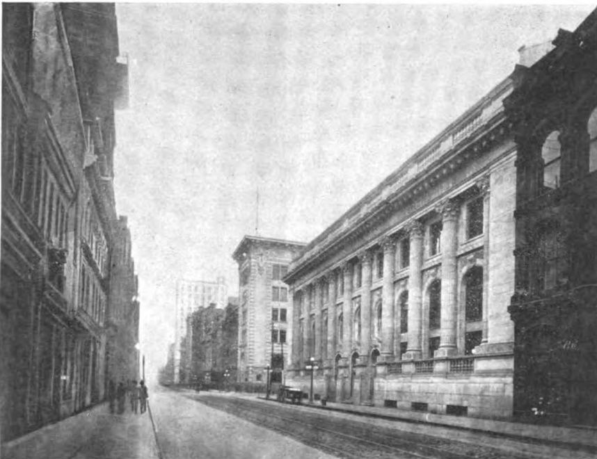
LOOKING EAST ON KING STREET
