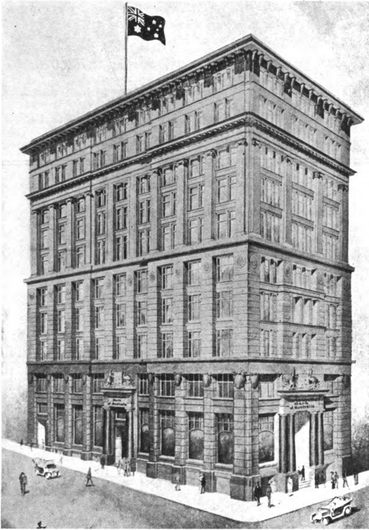
HEAD OFFICE BUILDING OF THE COMMONWEALTH BANK NOW IN COURSE OF CONSTRUCTION AT SYDNEY, N. S. W.
