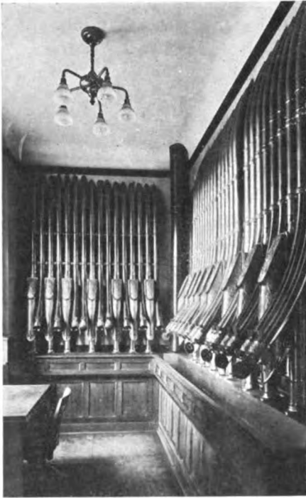
CENTRAL EXCHANGE FOR PNEUMATIC TUBES AND TELEPHONES
