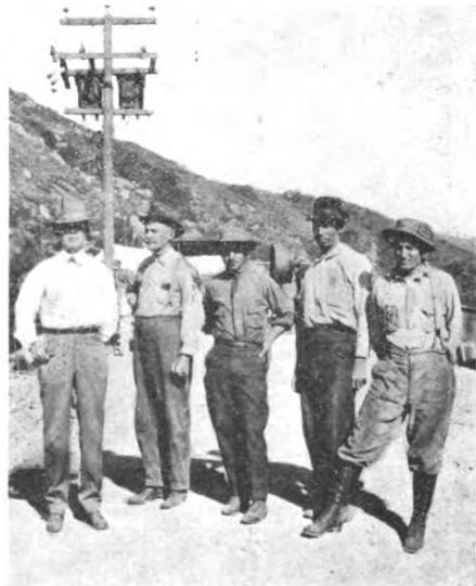
PART OF THE EXECUTIVE FORCE HANDLING THE WORK AT CAMP NO. 4.
