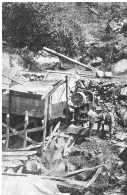
CONCRETE MIXER AND ROCK CRUSHER PLANT AT THE LOWER END OF TUNNEL NO. 12
