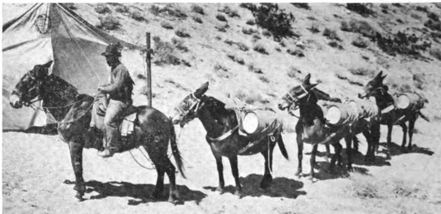
AT THE OUTLET, MANY MILES OF THE AQUEDUCT ZONE WERE INACCESSIBLE. IN THE CONSTRUCTION OF ROADS THESE SURE-FOOTED BEASTS OF BURDEN WERE EMPLOYED TO CARRY WATER, PROVISIONS AND DYNAMITE FOR BLASTING, AS SHOWN IN THE ILLUSTRATION.
