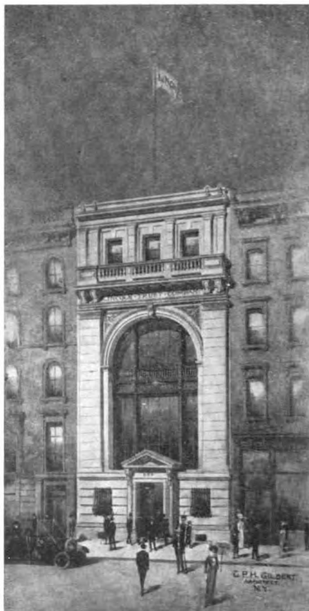
BUILDING OF THE LINCOLN TRUST COMPANY, NEW YORK, IN COURSE OF CONSTRUCTION.
