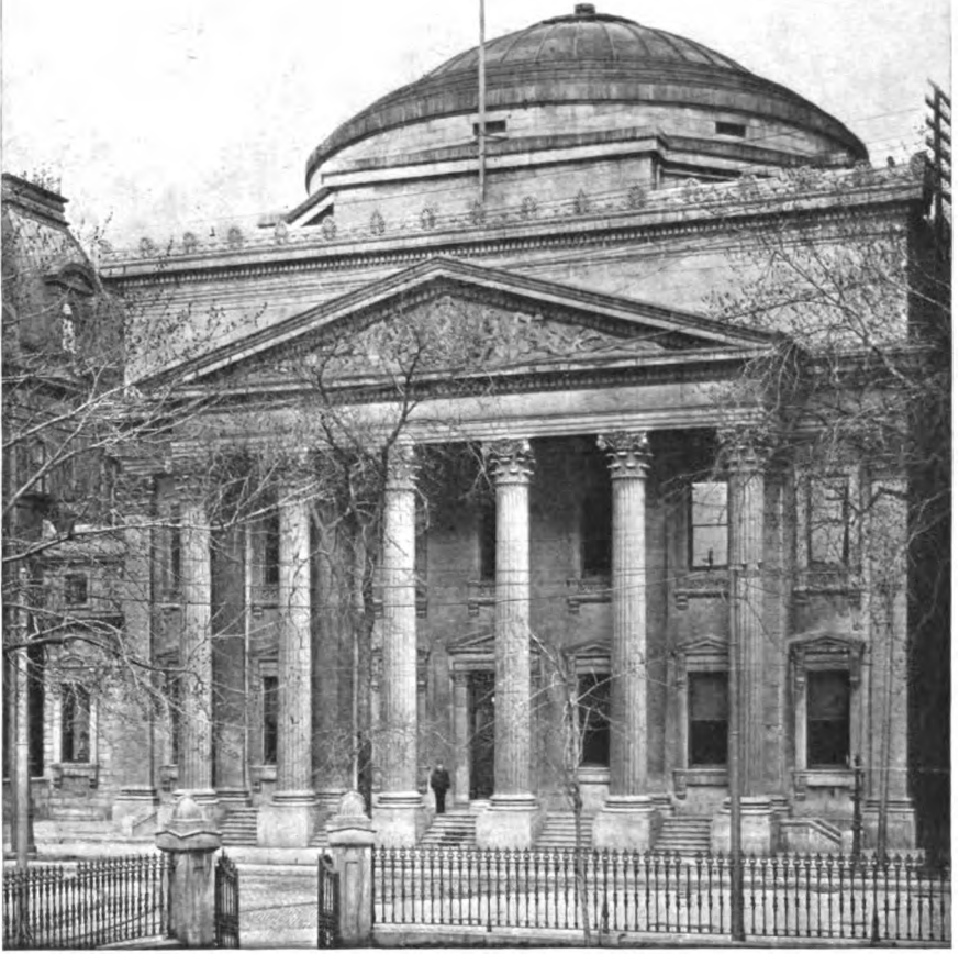
BANK OF MONTREAL—HEAD OFFICE, MONTREAL
