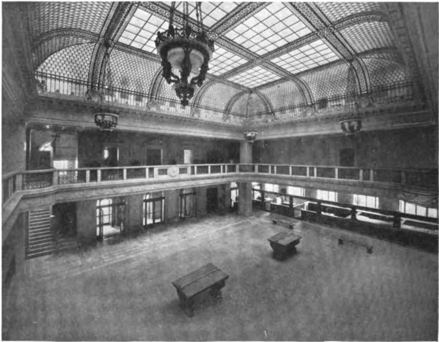
BANKING ROOM, LOOKING TOWARD MAIN ENTRANCE
