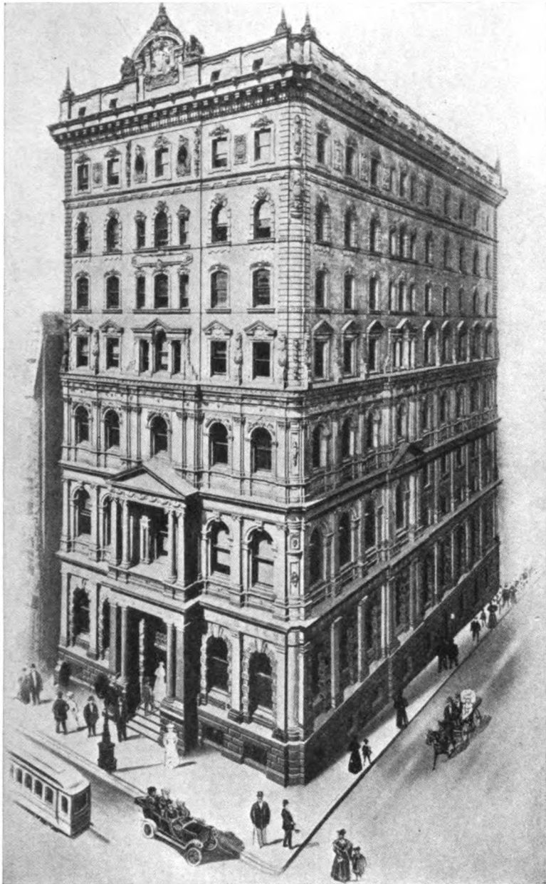
MERCHANTS BANK OF CANADA—HEAD OFFICE, MONTREAL
