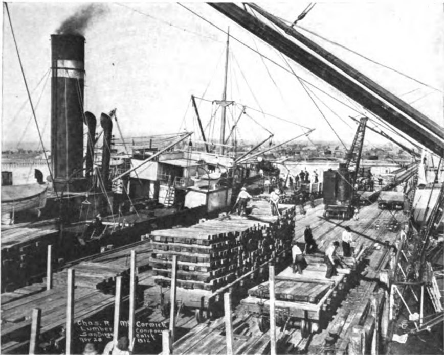
SAN DIEGO, CAL.—UNLOADING TIES—MCCORMICK LUMBER COMPANY'S WHARF
