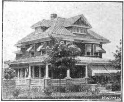
Residence of Mrs. Kircher, Lancaster, Pa. Covered with J-M Transite Asbestos Shingles.
