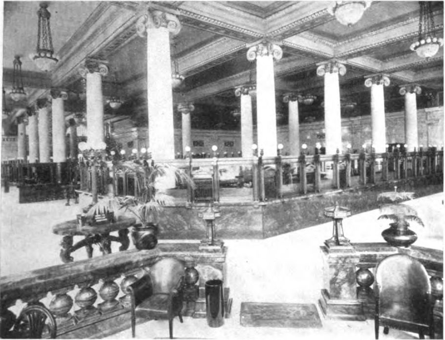
MAIN BANKING ROOM
