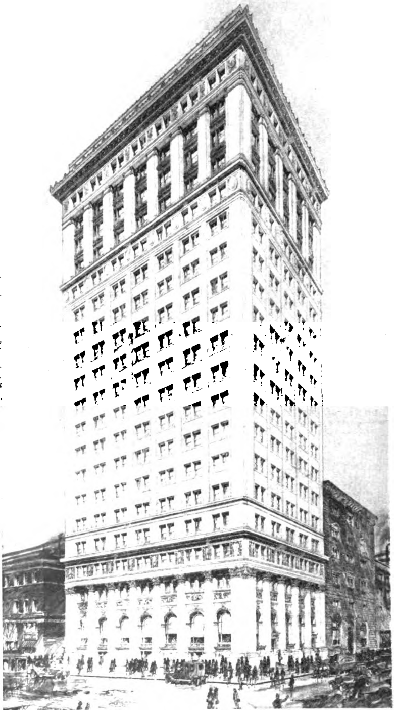
ROYAL BANK OF CANADA NEW BUILDING IN COURSE OF CONSTRUCTION AT TORONTO
