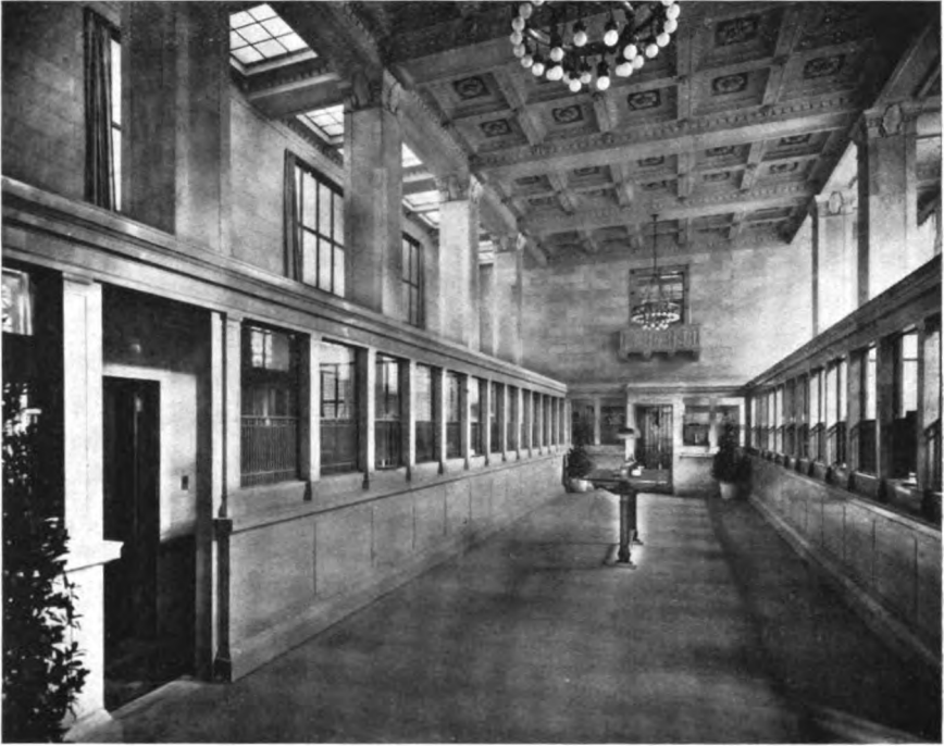
LOBBY, LOOKING TO REAR
