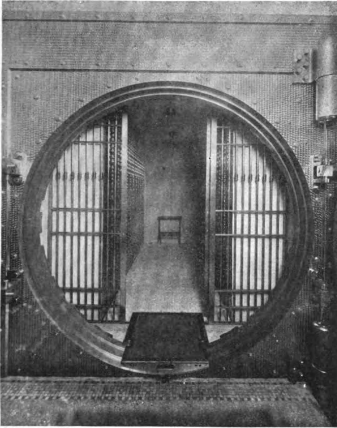
ENTRANCE TO SAFE DEPOSIT VAULTS UTICA TRUST AND DEPOSIT COMPANY
