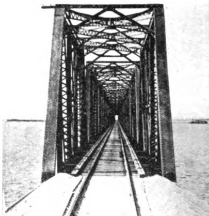
APPROACH TO THE BAHIA HONDA TRESTLE
