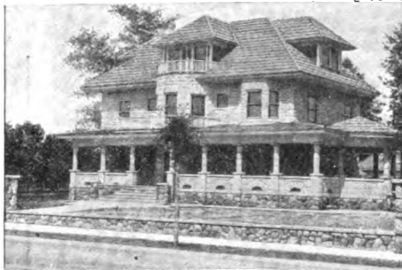
Residence of Mrs. Clara F. Taylor, De Land, Florida Roofed with J-M Asbestos Shingles.
