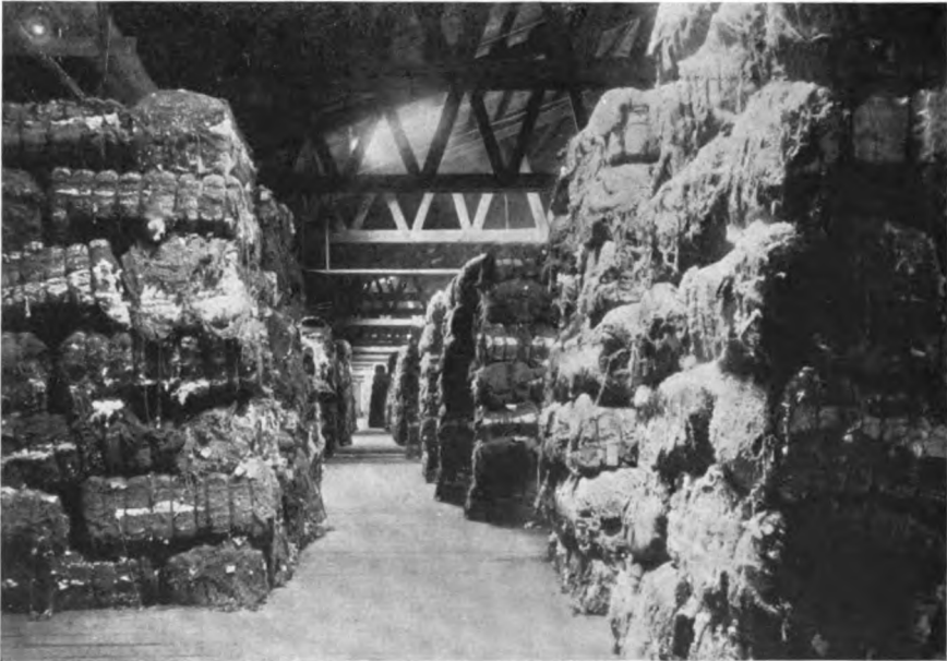
COTTON STORAGE ON SECTION OF AMERICAN DOCK PIERS, SHOWING SPACE OCCUPIED BY 6,000 BALES, ALL PROTECTED BY AUTOMATIC SPRINKLERS
