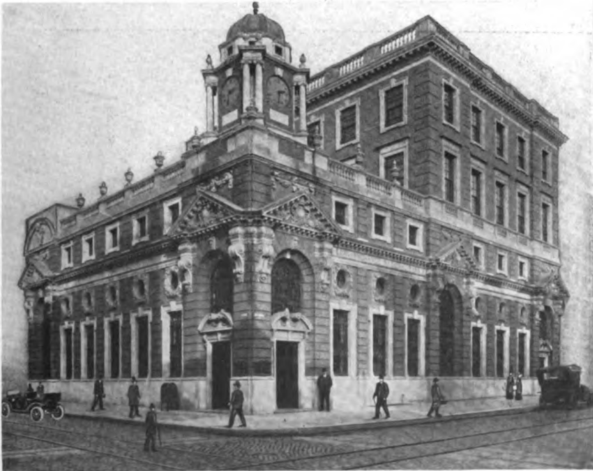
ENLARGED BUILDING OF THE CORN EXCHANGE NATIONAL BANK, PHILADELPHIA The lower portion was built in 1901; the higher part, including the first floor, is the addition completed in January, 1914.
