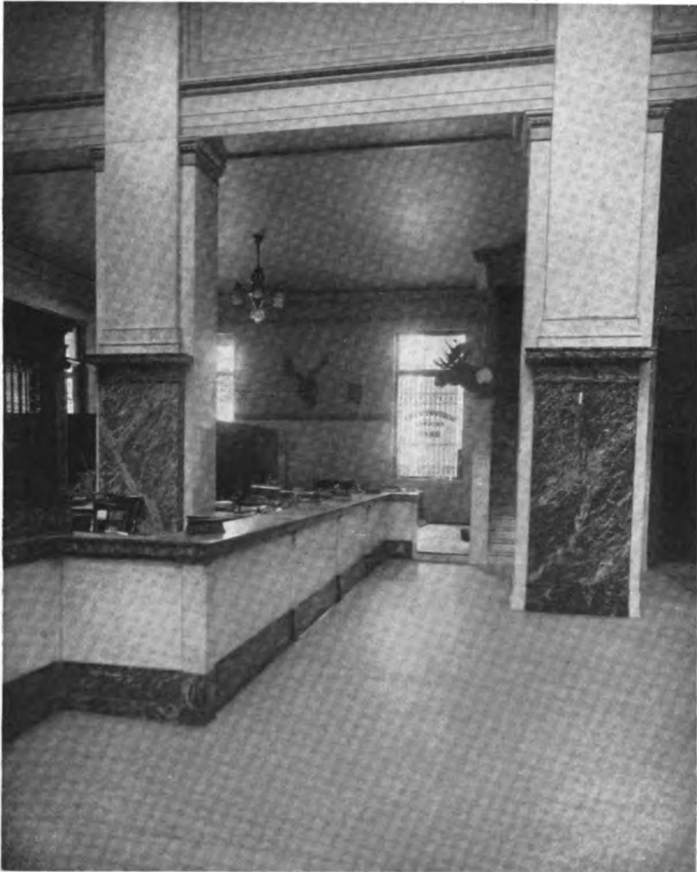
LOOKING TOWARD OFFICERS' QUARTERS NORTHWESTERN NATIONAL BANK, MINNEAPOLIS, MINN.
