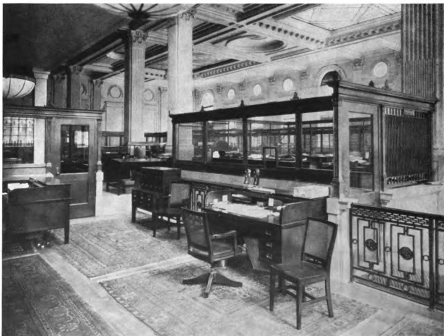
VIEW OF FIRST FLOOR CLERKING SPACE FROM THE OFFICERS' ROOM
