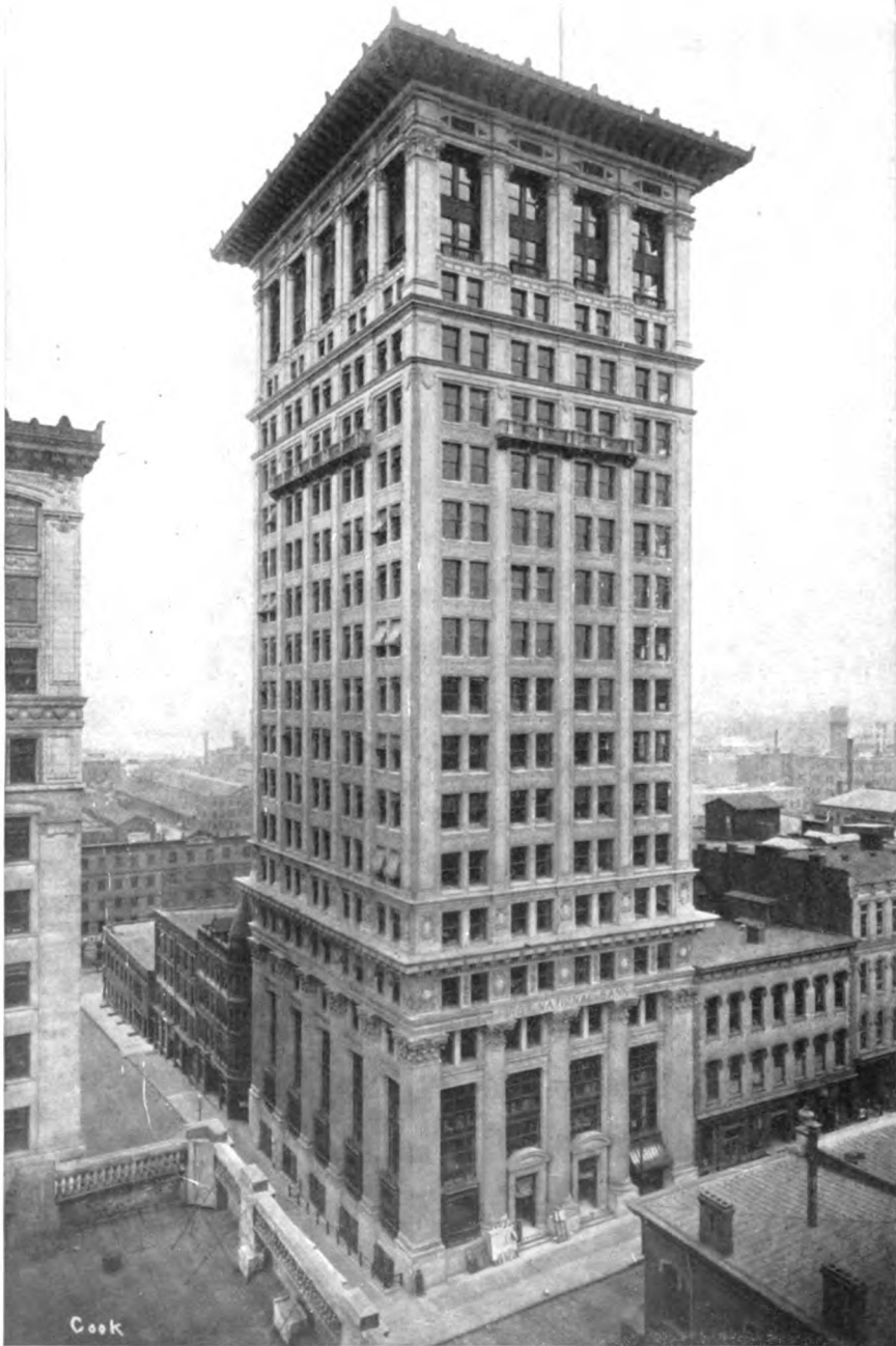
CHESAPEAKE & OHIO GENERAL OFFICE BUILDING, RICHMOND, VA.
