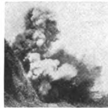
A DYNAMITE BLAST IN CULEBRA CUT
