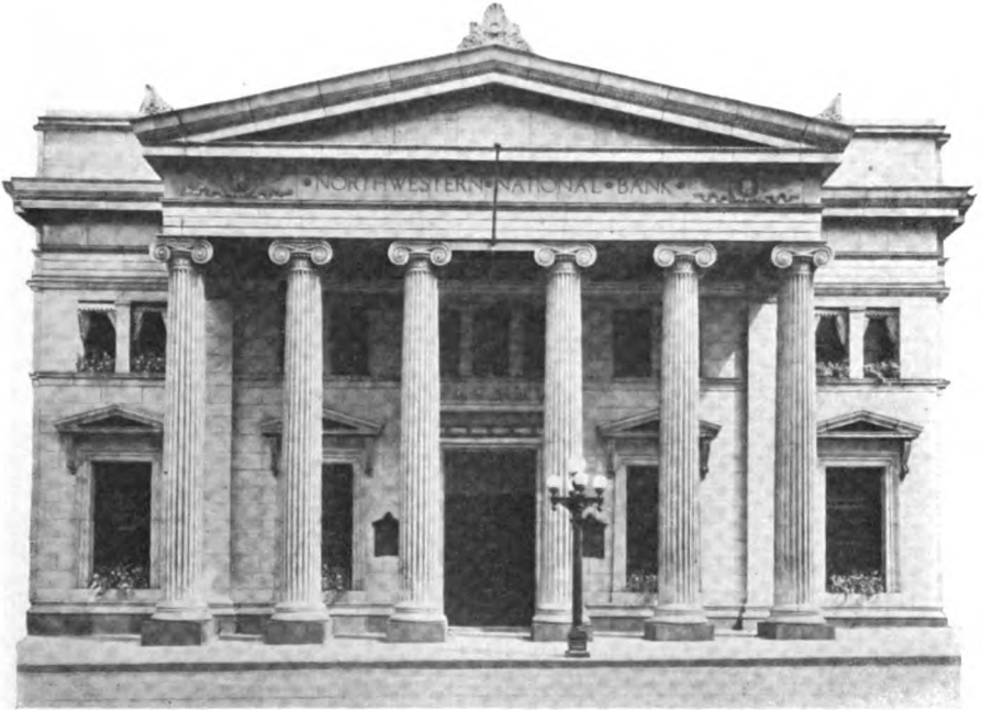
NORTHWESTERN NATIONAL BANK. MINNEAPOLIS, MINN.
