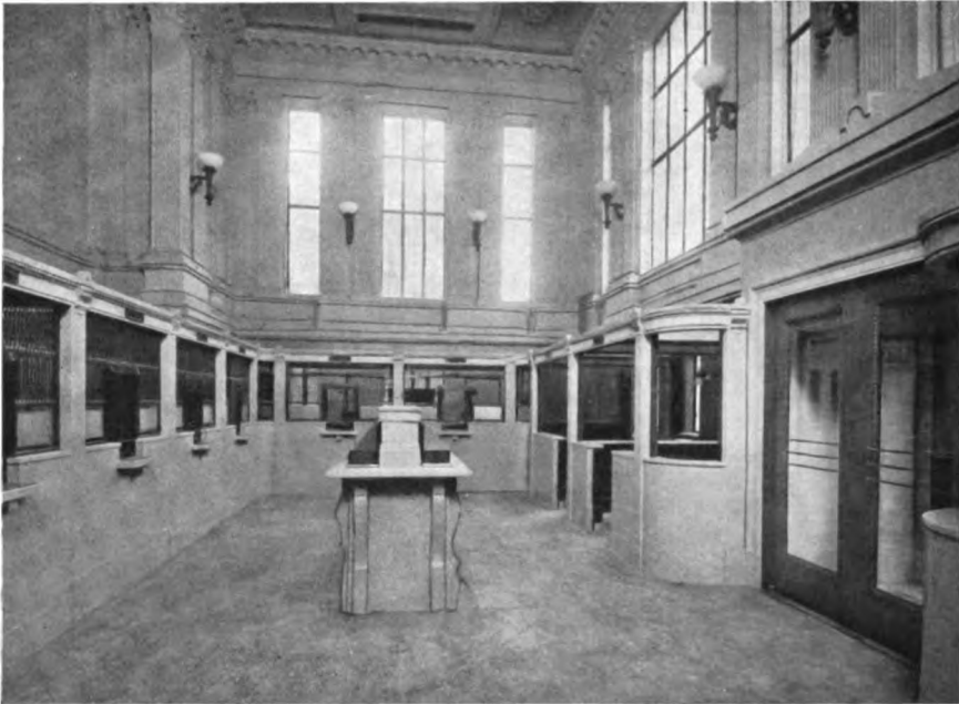
ANOTHER VIEW OF THE MAIN BANKING ROOM MANSFIELD SAVINGS BANK, MANSFIELD, OHIO
