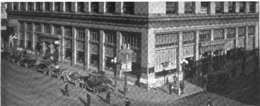
EIGHT DISPLAY CABINETS MAY BE COUNTED IN THIS PICTURE. GERMAN-AMERICAN TRUST AND SAVINGS BANK, LOS ANGELES, CAL.
