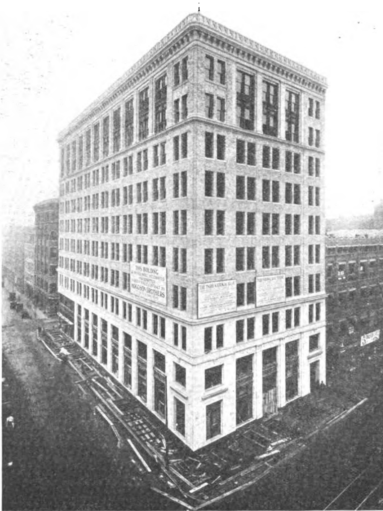
THIRD NATIONAL BANK BUILDING, SPRINGFIELD, MASS., NOW NEARING COMPLETION —AN EXAMPLE OF A SPLENDID TYPE OF COMBINATION BANK AND OFFICE BUILDING BEING ERECTED UNDER THE HOGGSON BUILDING METHOD
