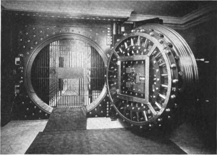
SECURITY VAULT. METROPOLITAN TRUST COMPANY, FIFTH AVENUE BRANCH
