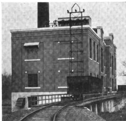
Williamsburgh Power Plant Penn Central Power and Transmission Co., Williamsburgh, Pa. This company is under Day & Zimmermann management
