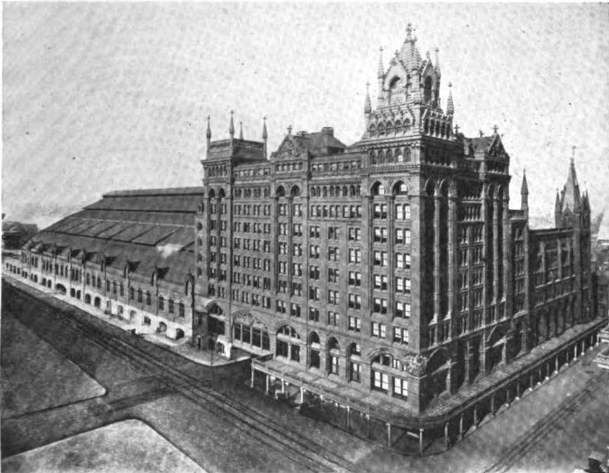
Broad Street Station, Pennsylvania Railroad;
