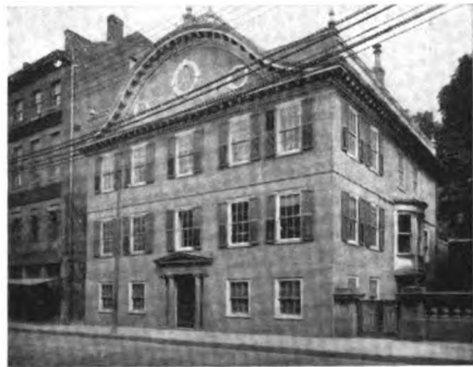
Colonial Mansion, built in 1774, Present Home of the Providence National Bank
