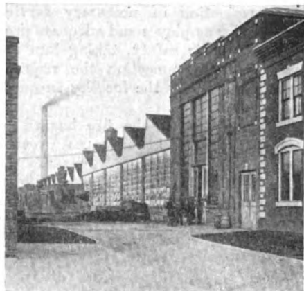
Plant of the Cincinnati Bickford Tool Co., Cincinnati, Ohio
