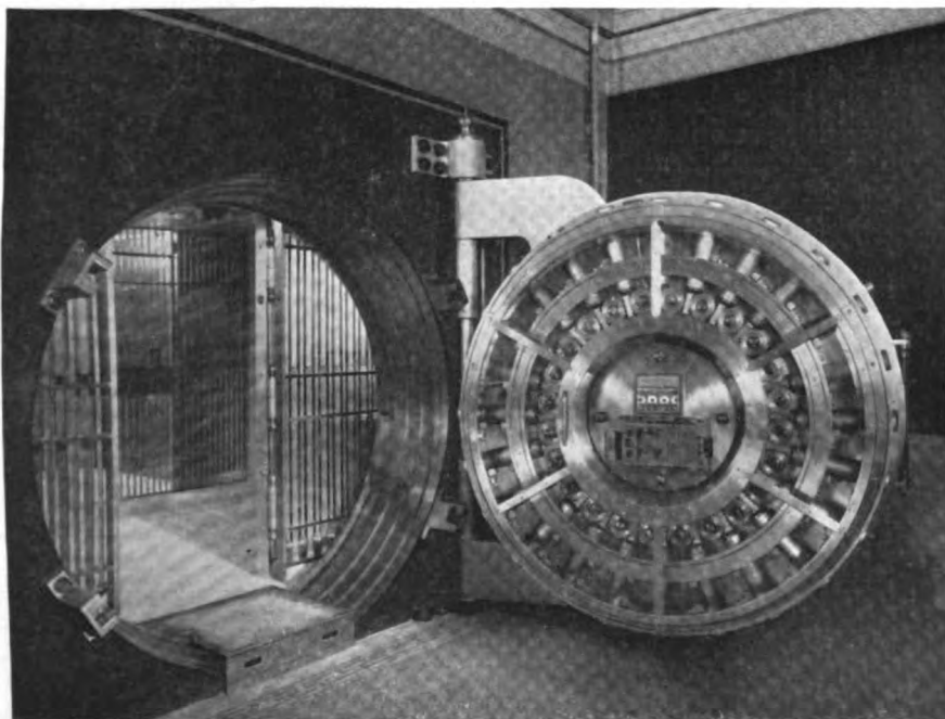
Exterior of Vault on Main Floor
