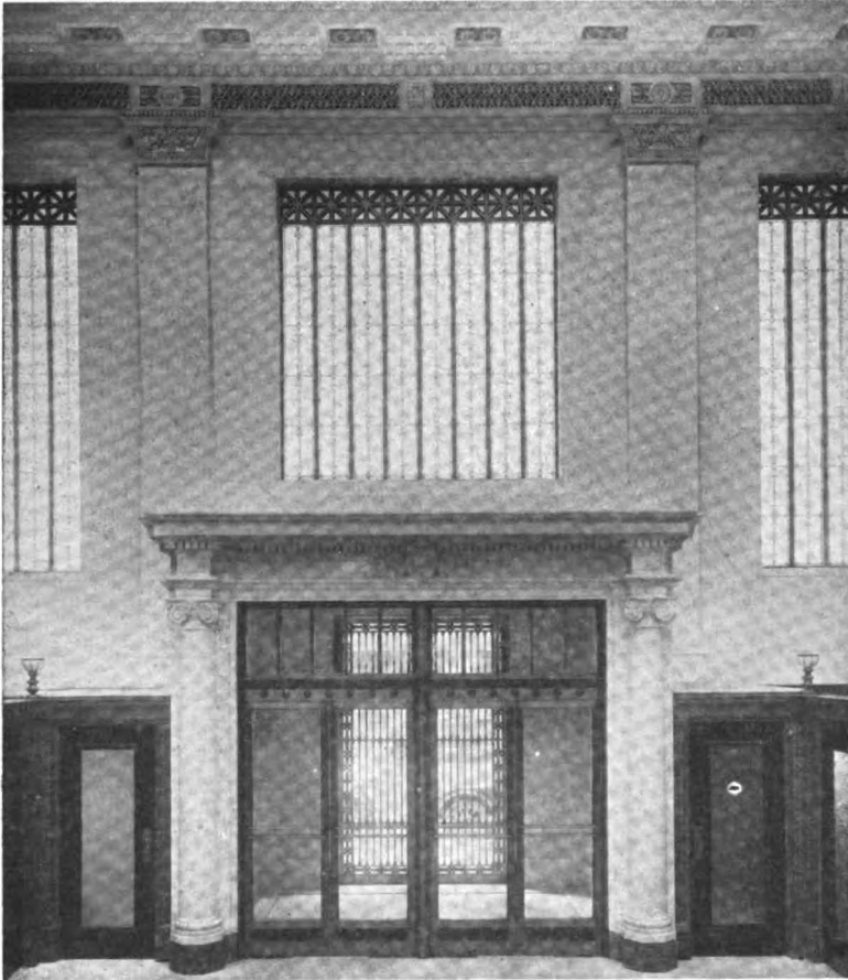
Main Entrance, Security National Bank, Los Angeles, Cal.
