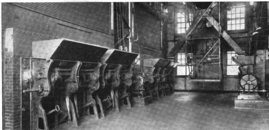
Williamsburgh Power Plant, Boiler Room, Showing Automatic Weighing Larry and Automatic Stokers
