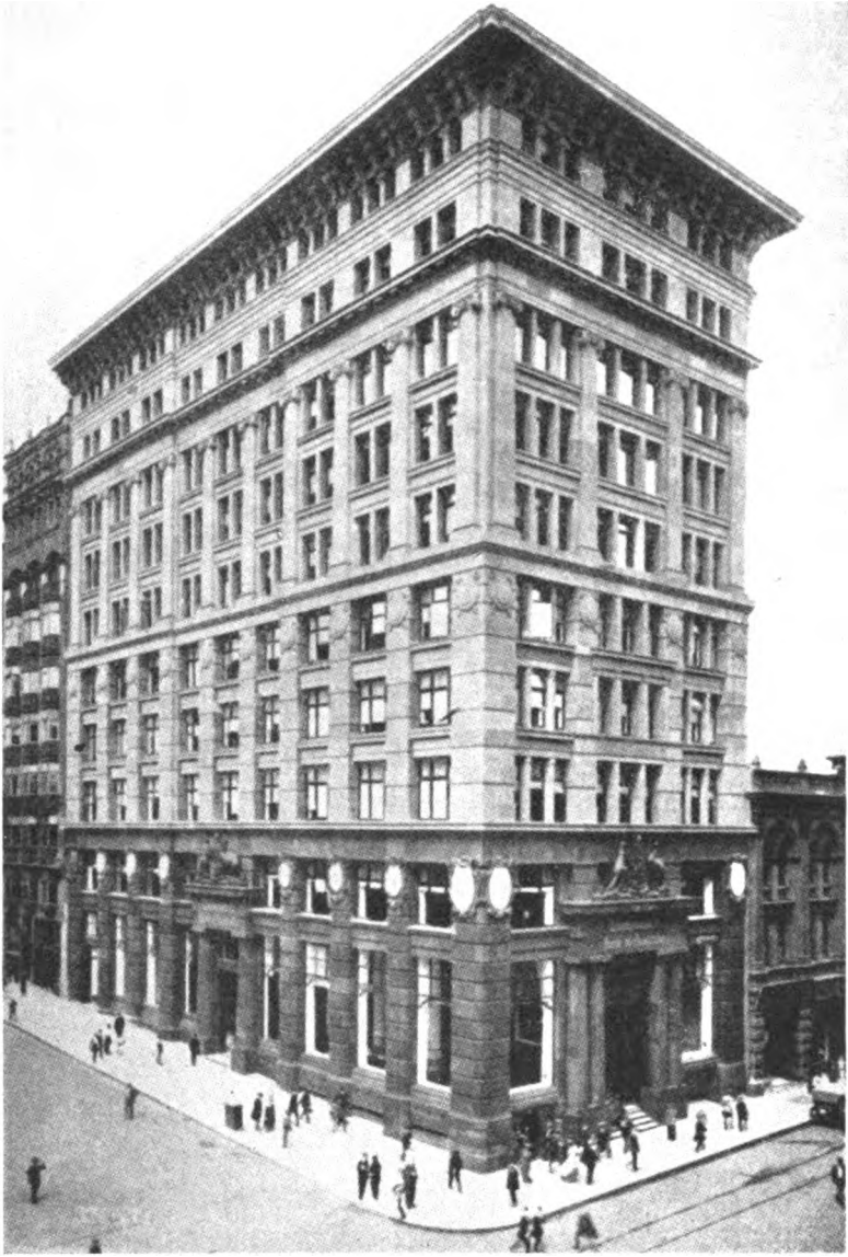
The Head Office. The Commonwealth Bank of Australia, Sydney, Australia
