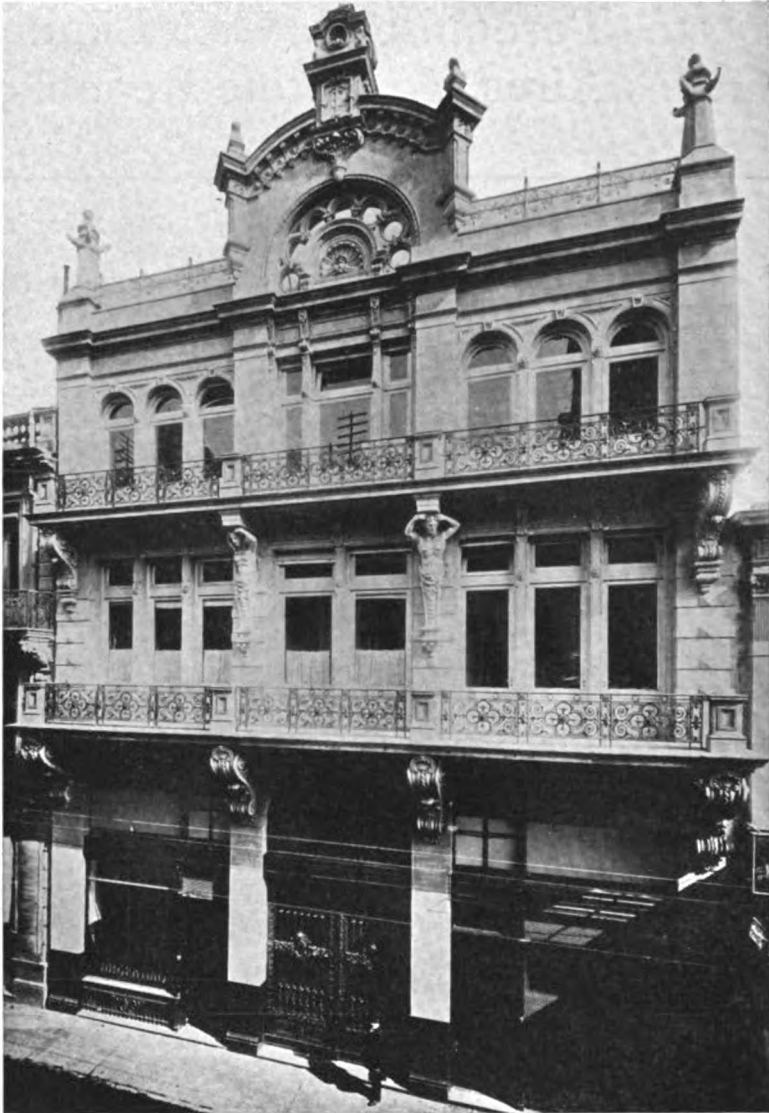
Tornquist Building, 132 San Martín, Buenos Aires
