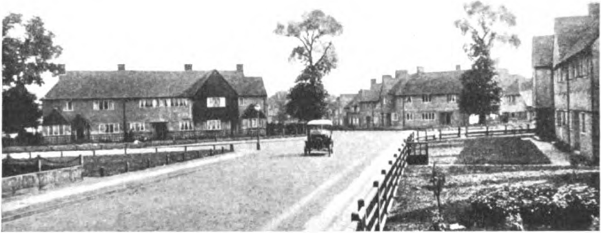
Government Housing Scheme, Well Hall, Woolwich, 1915. Congreve Road (Boughton Road Crossing) Looking South
