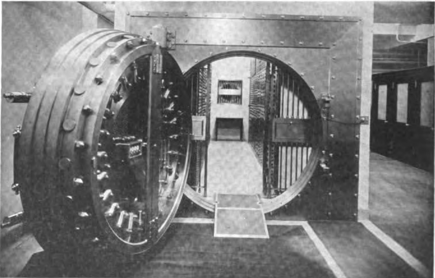
Twenty-five Ton Vault Door Open, Interior View Showing Section of Safe Deposit Box and Emergency Door in Rear
