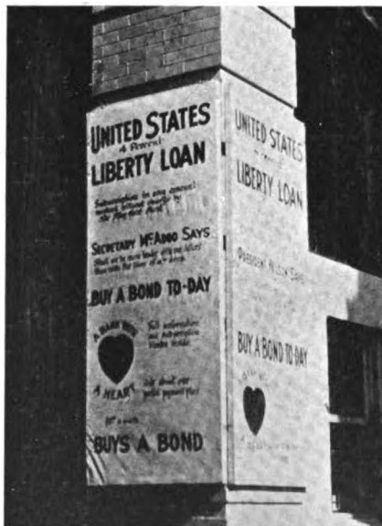
Corner of the Bluefield (W. Va.) Bank Building during the Liberty Loan Campaign
