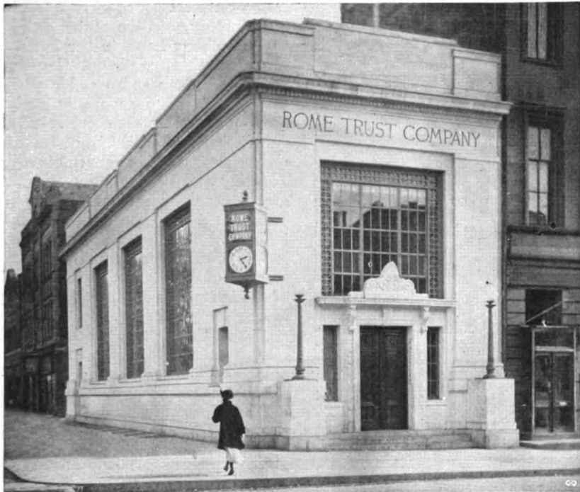
Indiana Limestone Banking Building of the Rome Trust Company, Rome, N. Y.
