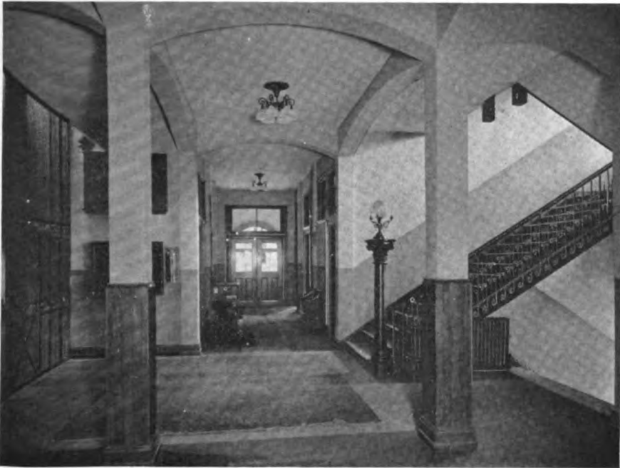
The Main Corridor on the First Floor
