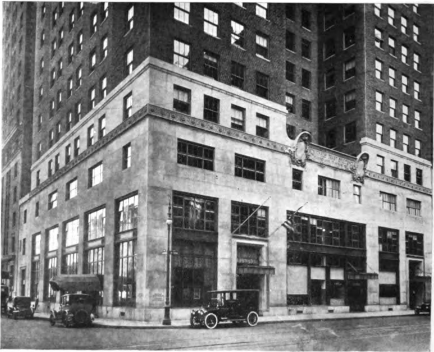
Equitable Trust Company, Uptown Building, 45th Street and Madison Avenue, New York
