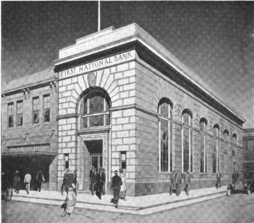
Distinctive individual Italian Renaissance bank building under construction by Hoggson Brothers, Builders, New York, Chicago and Atlanta, for the First National Bank of Bryan, Texas
